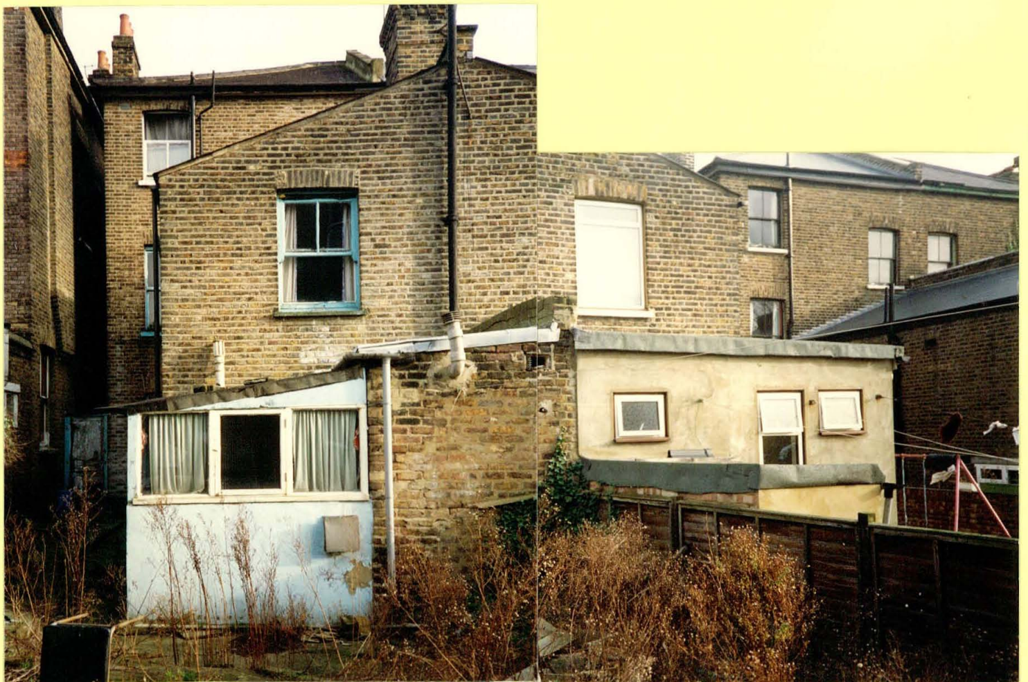
rear of no. 52
