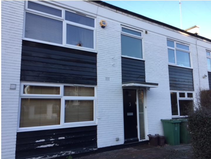
Photo 1 (above): Front elevation of 106 King Henry's Road
