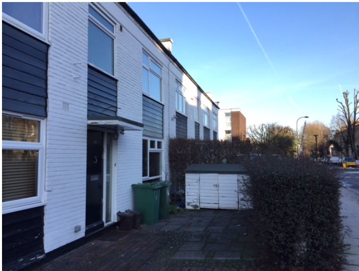
Photo 2 (above): Front elevation of 106 King Henry's Road looking east
