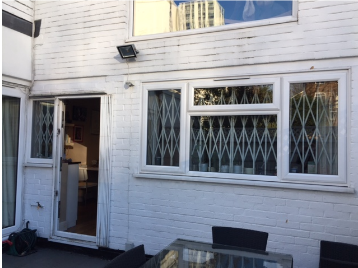
Photo 10 (above): Ground floor rear elevation of 106 King Henry's Road
