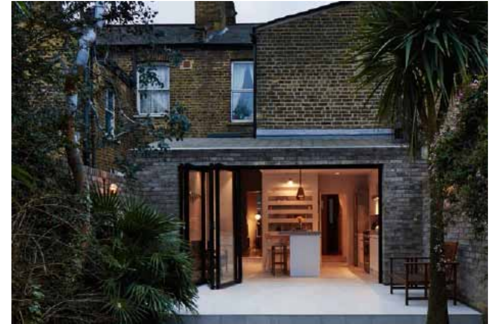
Visually contrasting brickwork
