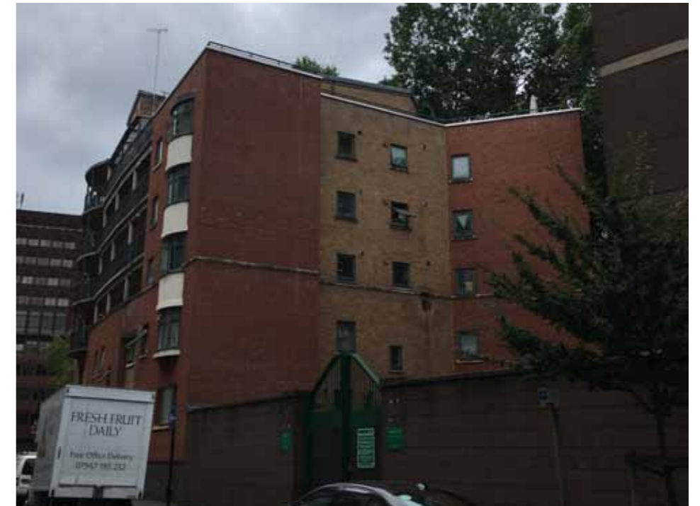
Streetview of Pendrell House (Looking South)
