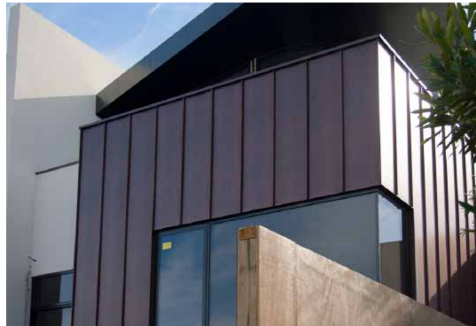
Dark copper colour standing seam zinc finish
