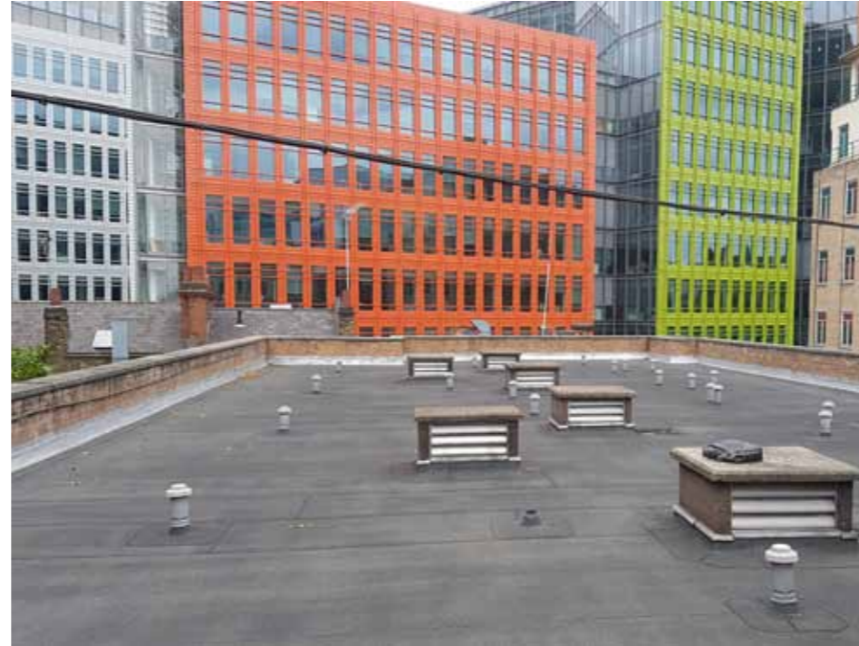
45 New Compton Street, Existing Rooftop
