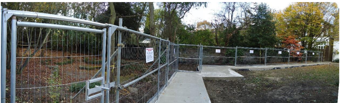
Figure 4. Photograph to illustrate installed protective fencing
