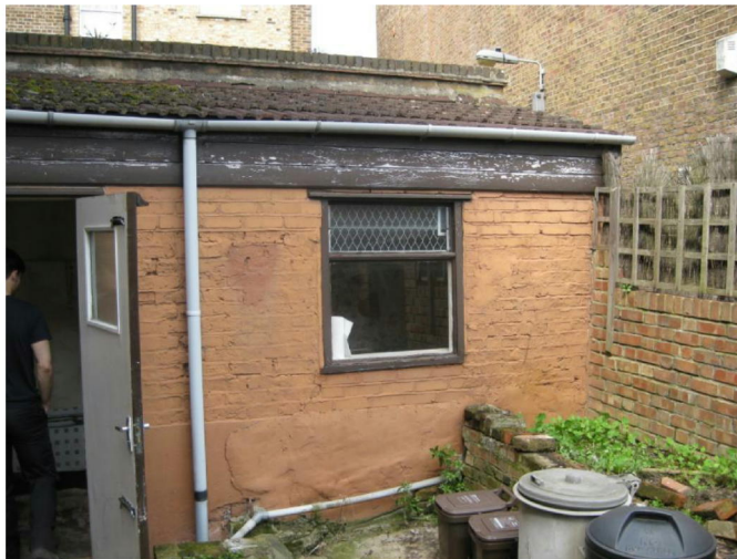
External view of Kitchen
