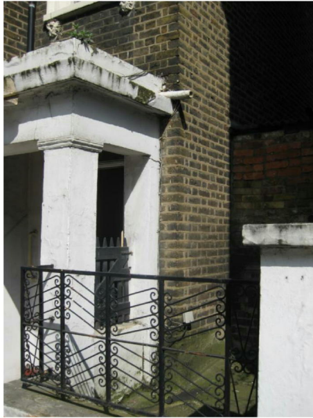
Existing metal railing to be replaced with period heritage railings
