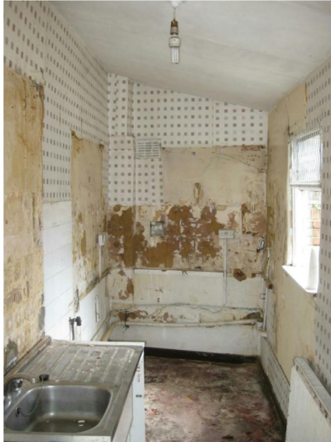
View into Kitchen (existing units removed)
