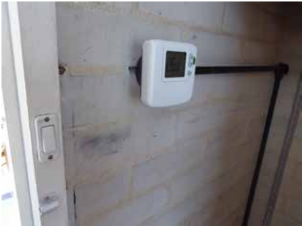
CONDUITS TO BE NEWLY INSTALLED, THERMOSTATS TO BE CONCEALED
