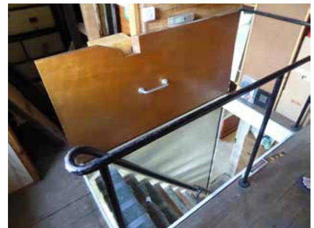
LANDING HATCH TO BE REMOVED AND NEW STUD WALL ERECTED FOR NEW BATHROOM AND BOILER CUPBOARD
