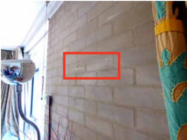
EXAMPLE OF DAMAGED BRICKWORK (TO HAVE PLASTERED FINISH)
