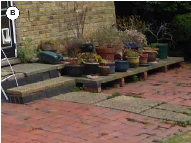
BRICK PAVERS TO BE LAID FLAT ON NEW SUBSTRATE
