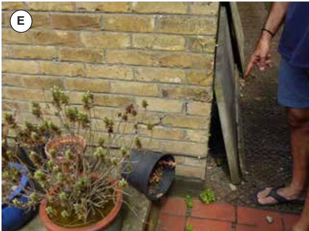
SUBSIDENCE TO BE REPAIRED - NEW POINTING TO MATCH EXISTING ONCE REMEDIED
