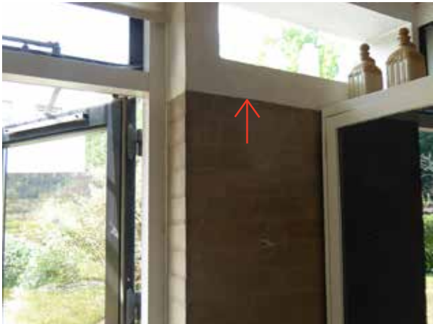
PROPOSED PLASTER FINISH TO STOP SHORT OF CONCRETE WINDOW DETAIL
