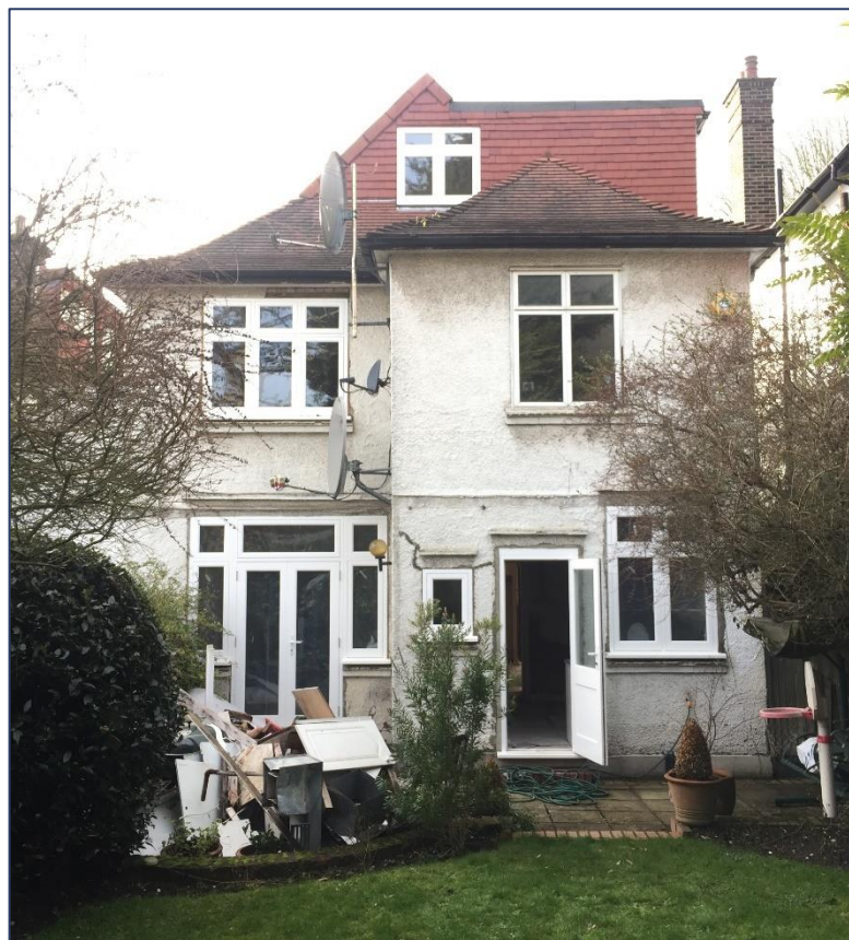
Fig. 5 – Existing rear extension
