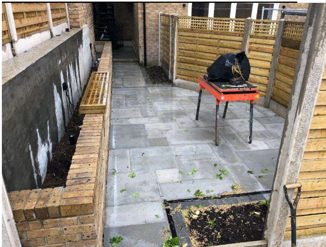
Soft landscaping to rear gardens
