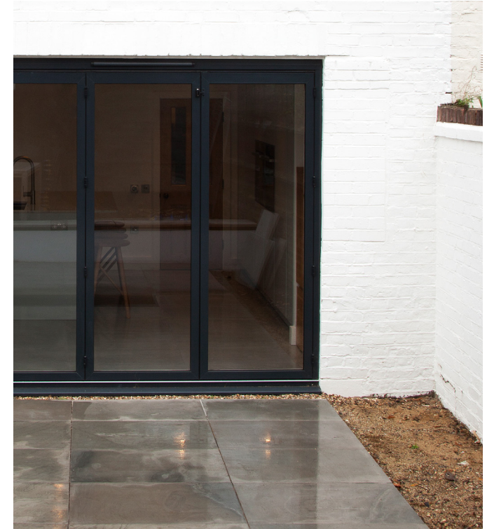
Metal frame openable glazing and stone paved patio
