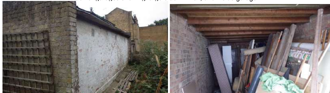
Back of garages showing large crack in wall, and inside garage 1
