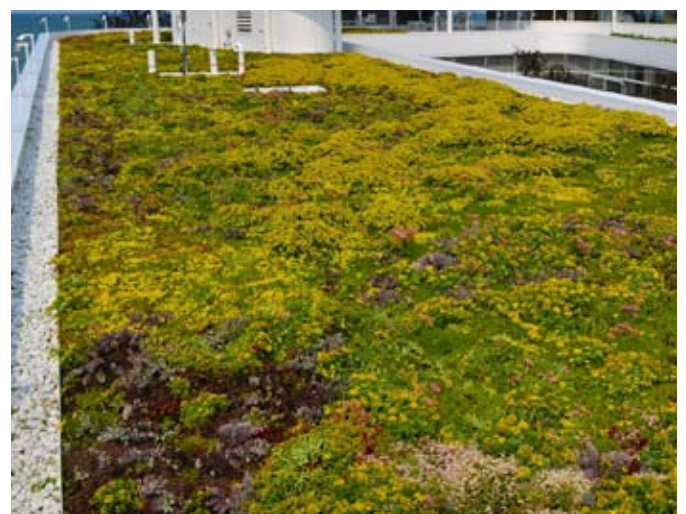
Biodiverse green roof to flat roofs which contribute to biodiversity and sustainable drainage
