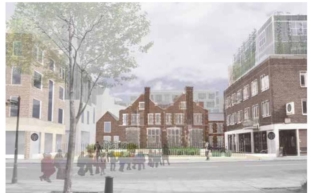
Toynbee Hall, Tower Hamlets
