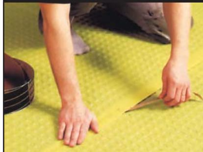
DELTA®-FM is specifically designed for floor applications, to combat dampness, and contamination. The special low stud profile (3mm) minimises changes in floor levels but still provides an air gap to achieve damp pressure equalisation.
