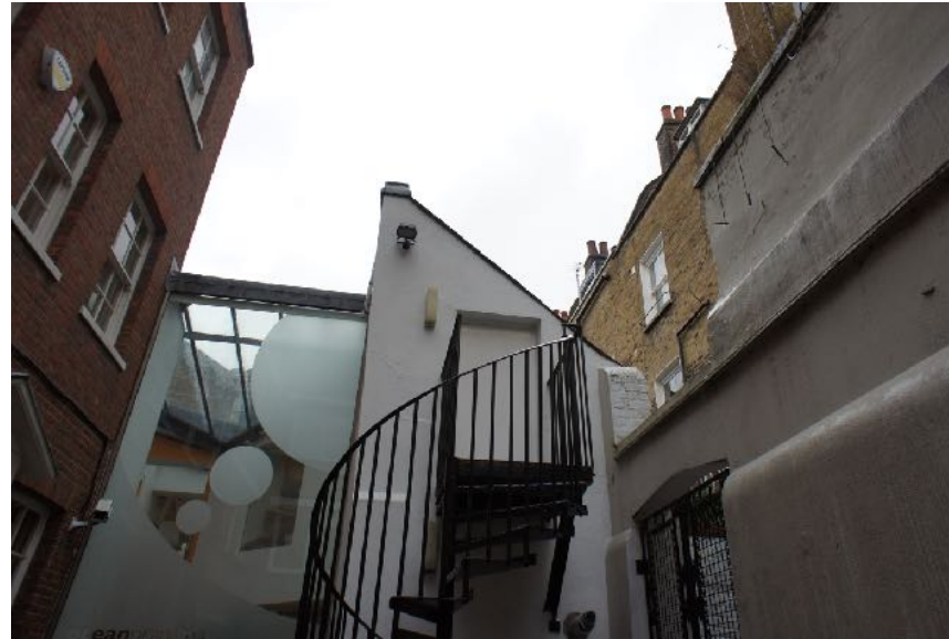
View looking at non compliant spiral escape stair at 3 Bromley Place.
