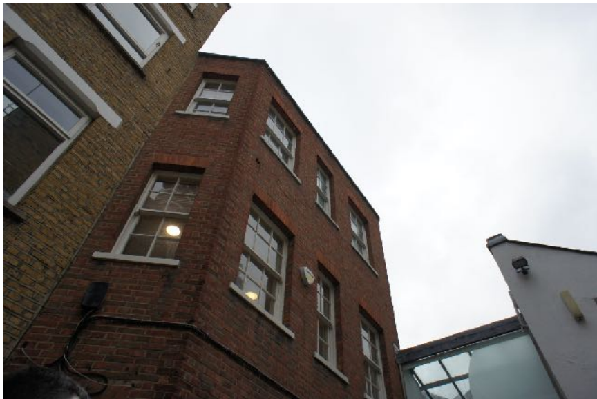
View looking up to townhouse that forms part of 3 Bromley Place.
