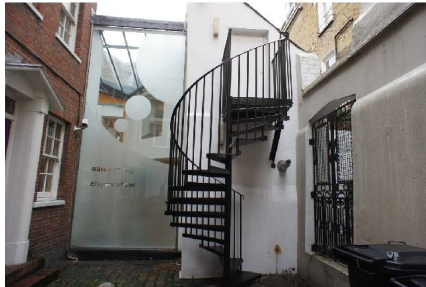
View looking at glazed screen that was formerly the entrance consented at 3 Bromley Place.
