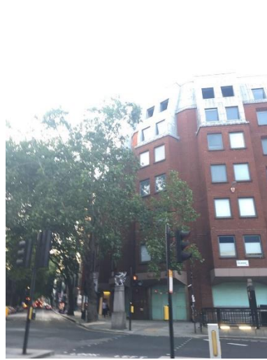
Photograph 2: South-western corner of 150 Holborn
