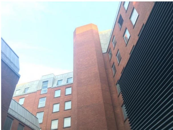
Photograph 3: Internal courtyard of 150 Holborn
