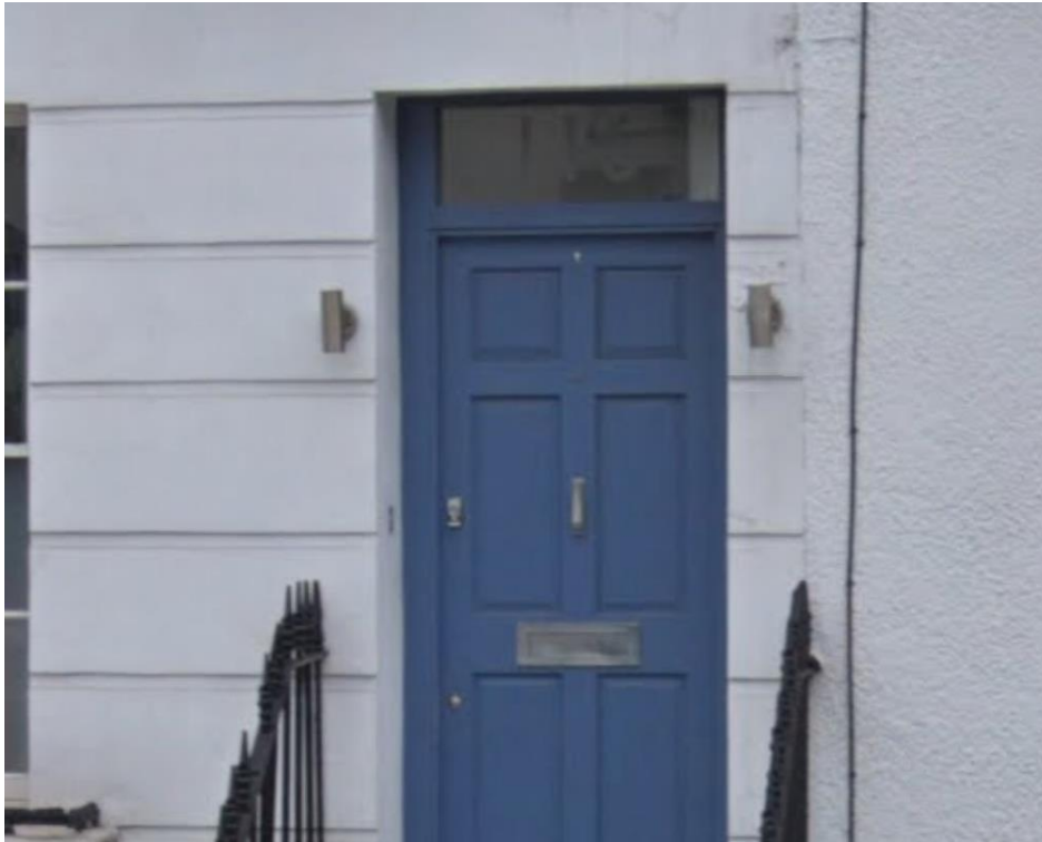
Fig. 5 Up-and-down lights at neighbouring 116 Prince of Wales Road
