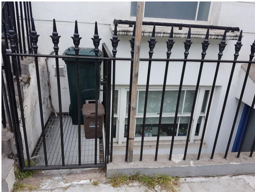
Fig. 4 Bin store at 116 Prince of Wales Road
