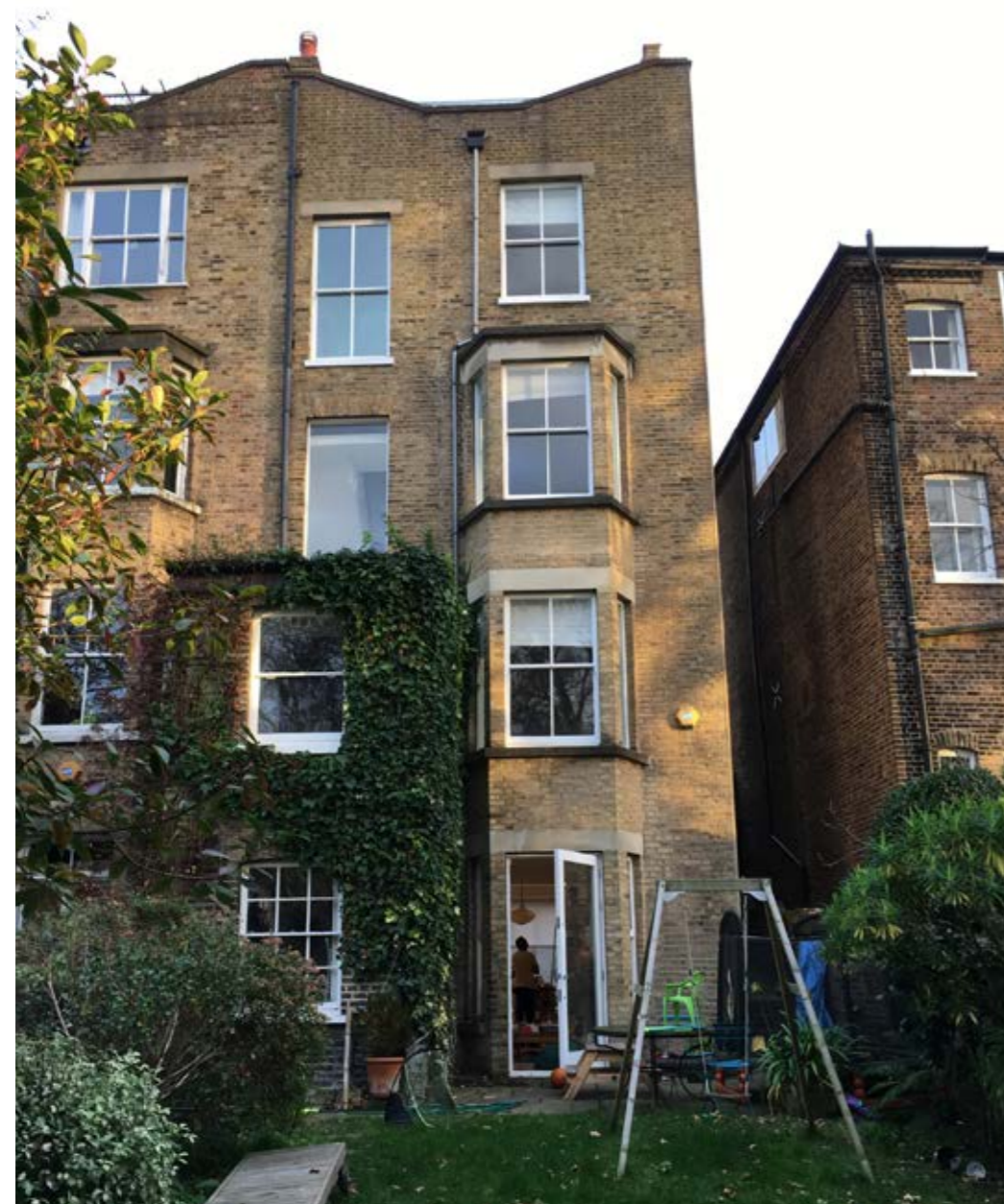
Rear view of 24 South Hill Park building from the rear.
