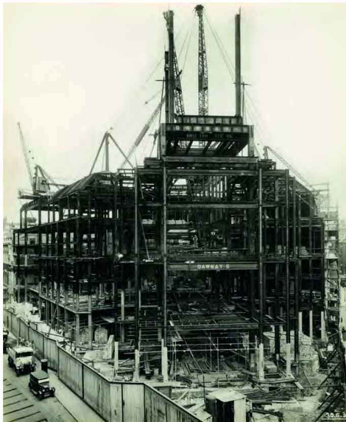
Figure 5: Western end in construction c1929 (©UGLE)
