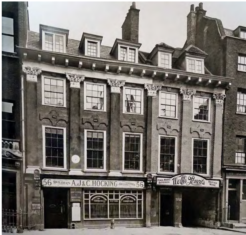
Figure 3: 55 & 56 Great Queen Street in 1908 – examples of buildings demolished to make way for Freemason's Hall in 1927 (© Historic England)
