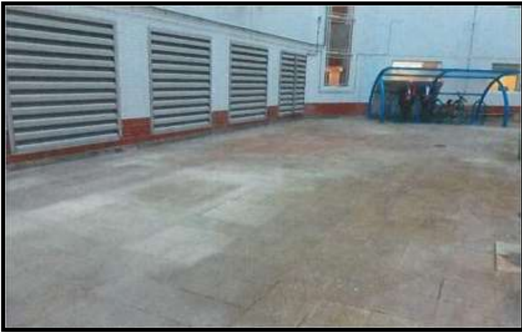
FREEMASONS' HALL PROPOSED LOCATION FOR STAND BY GENERATOR
