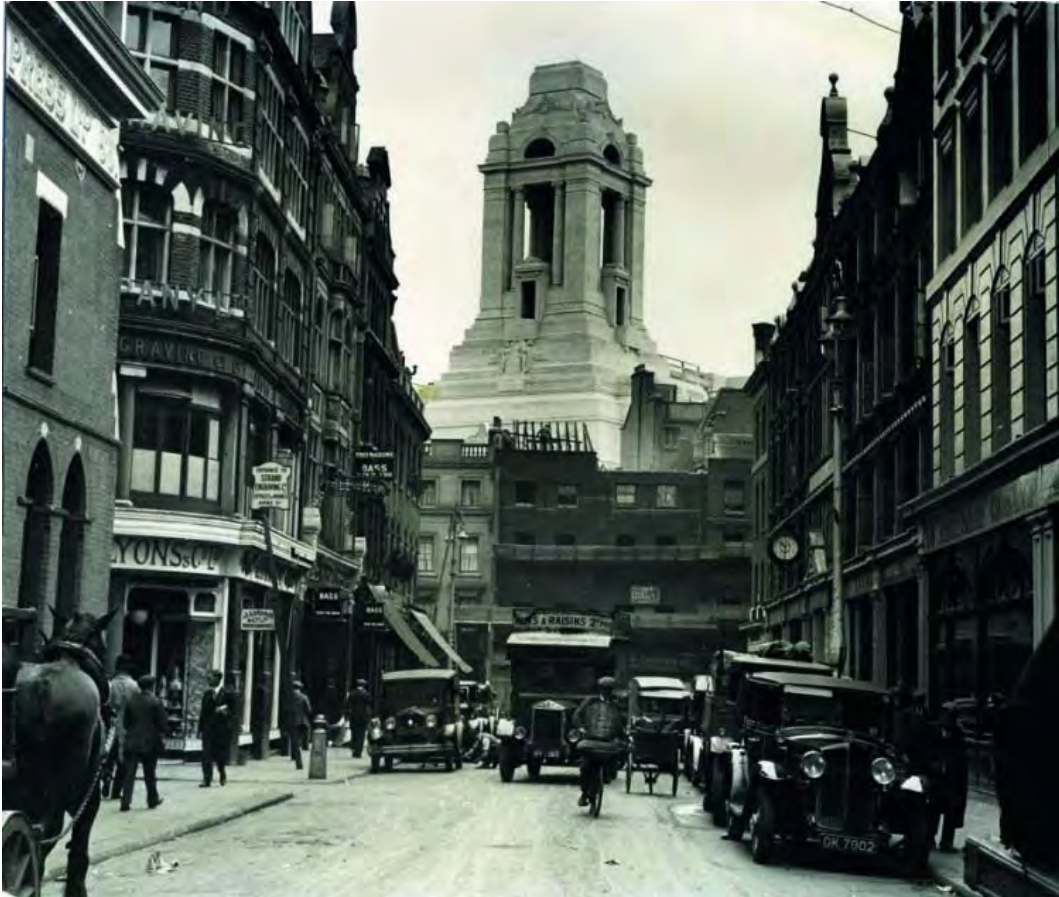
Figure 7: View over partially demolished buildings 1931 (©UGLE)
