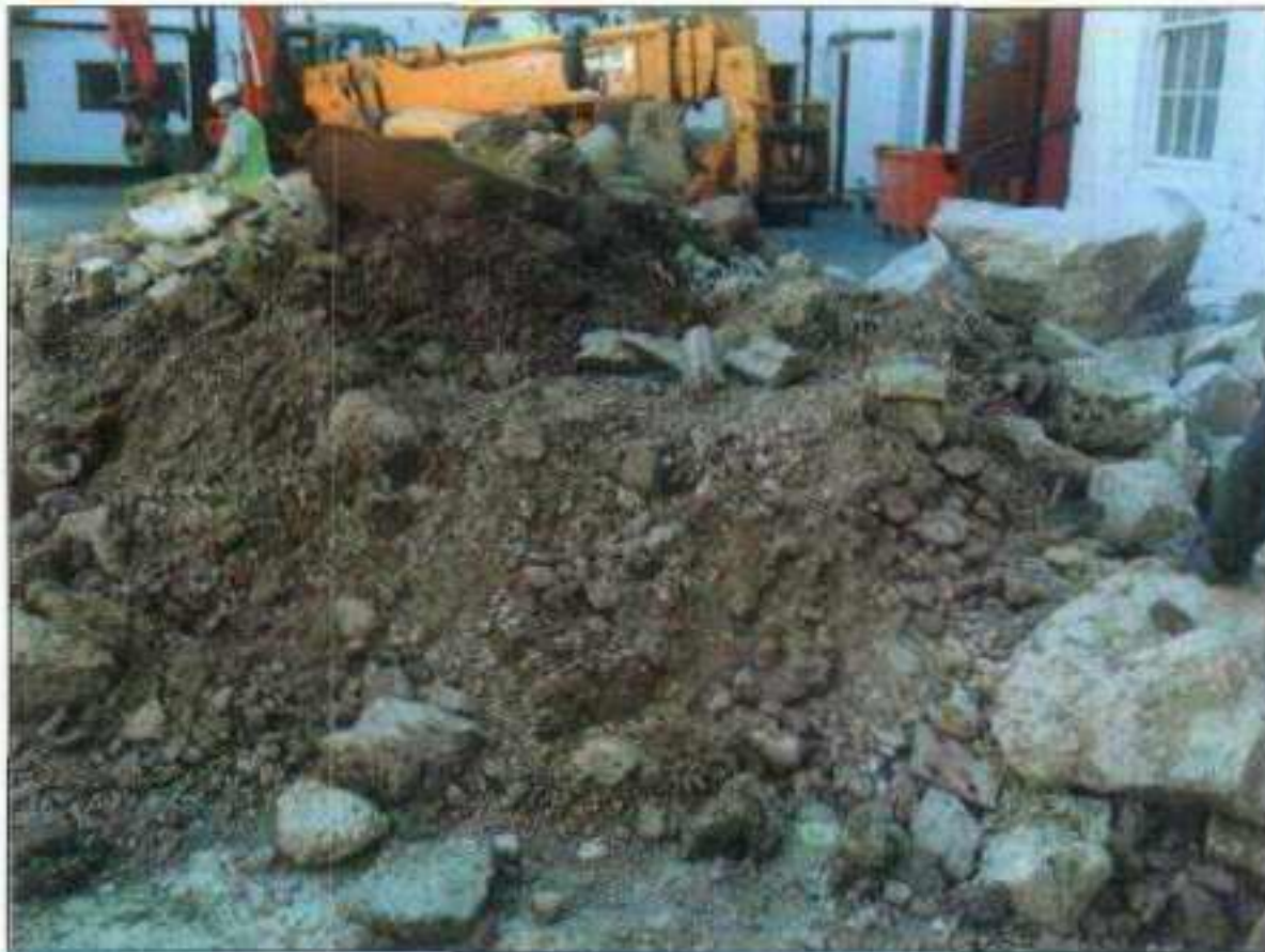
Photo 6. STP01 – Excavated material for re-use
