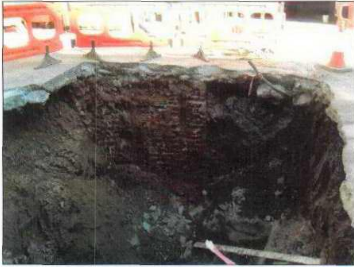
Photo 1. Face of excavation looking north
