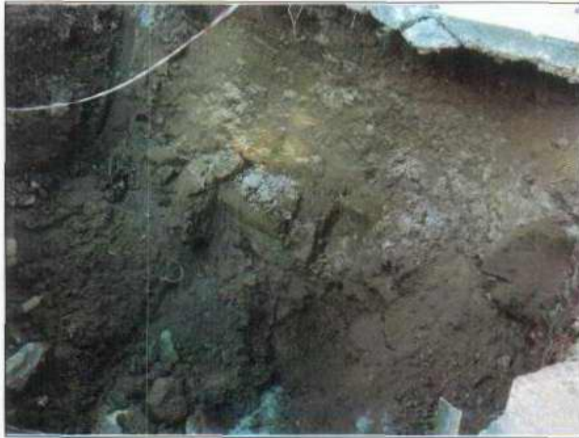
Photo 2. Western face and base of excavation
