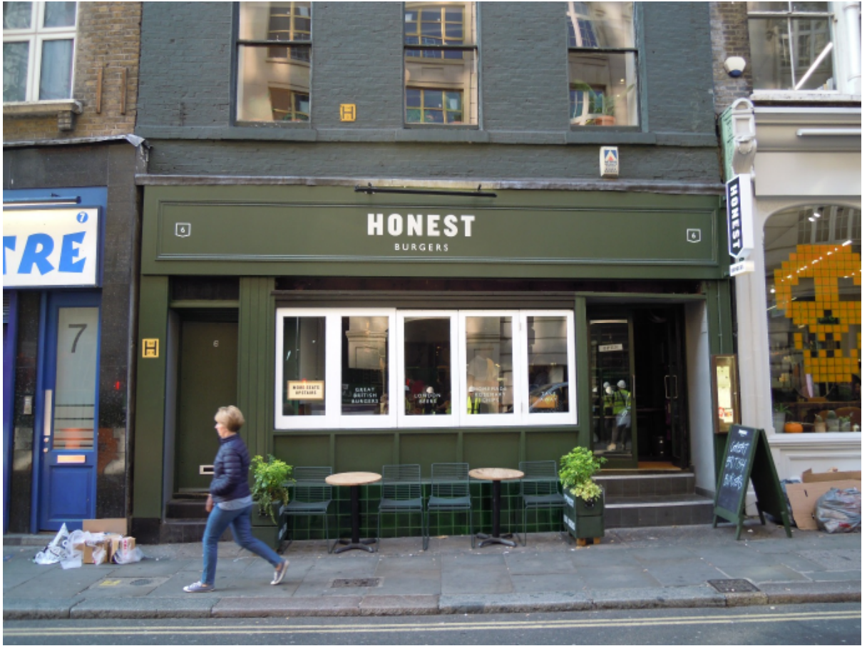
Shopfront and adverts now installed
