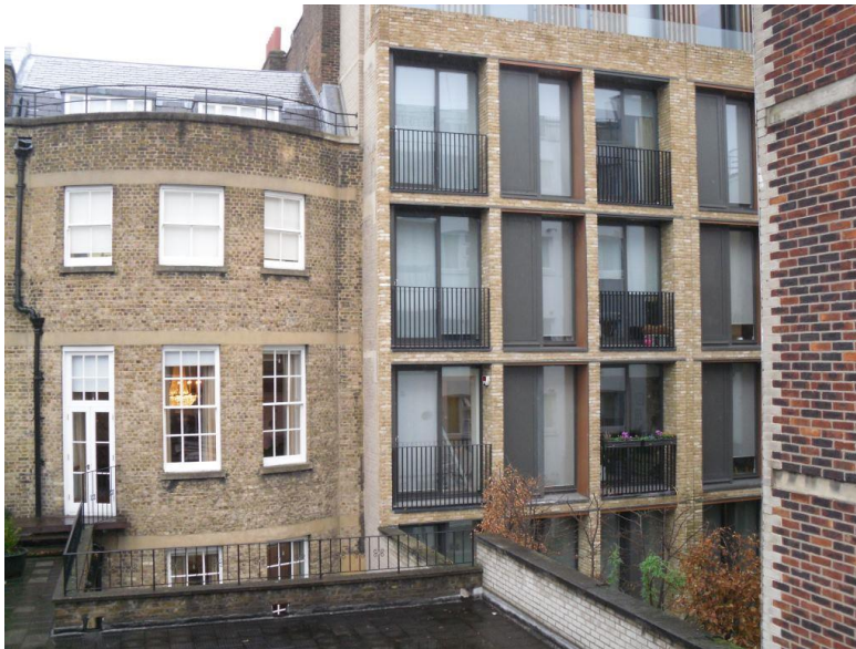
Rear view nos.30; 31-33 John St.
