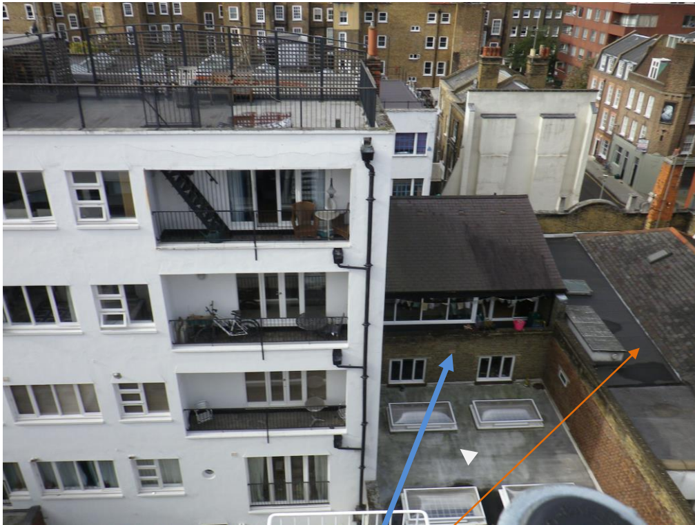
View due north-west R/O nos. 29- 31; 27 & 25 John's Mews
