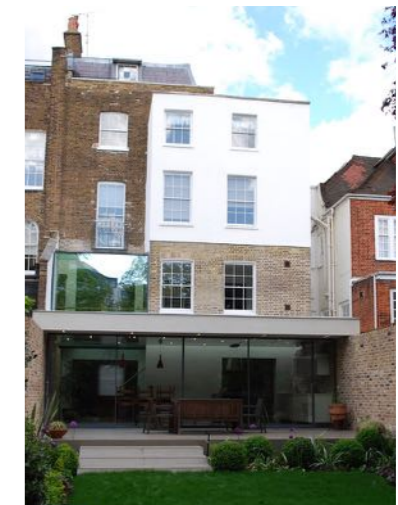
Hamilton Terrace, NW8 - Extension & modernisation of grade II listed terrace house.
