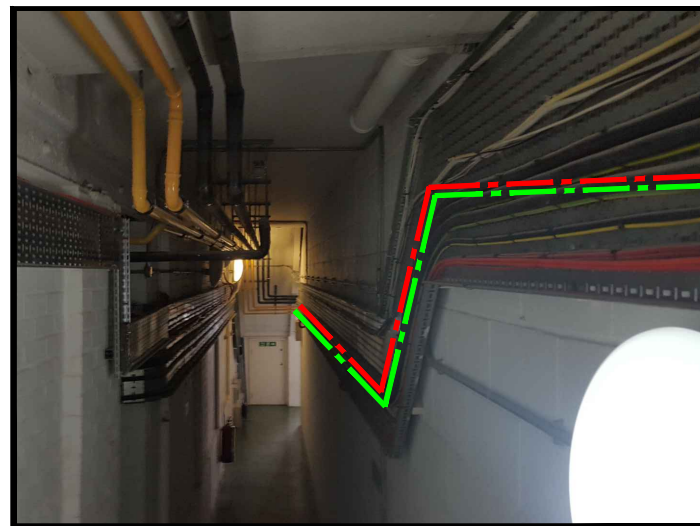
EXISTING POWER & CPC EARTH CABLE ROUTE 4
