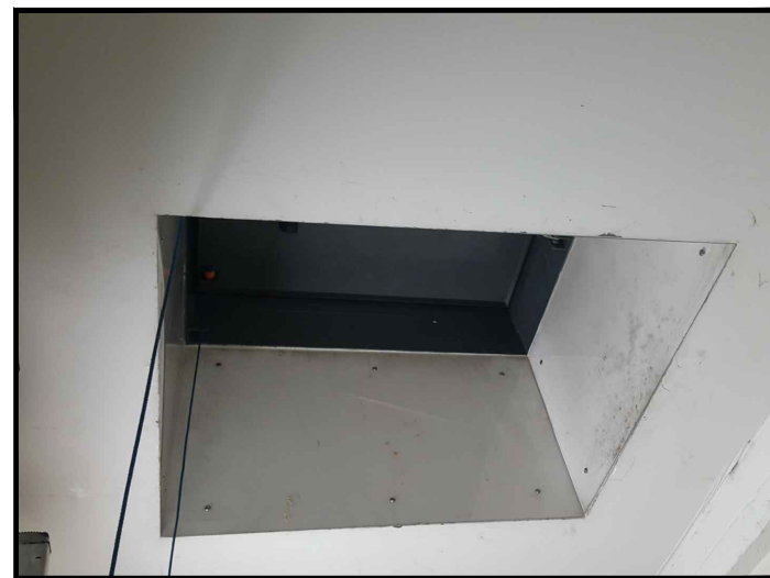
EXISTING ACCESS HATCH IN THE ROOF
