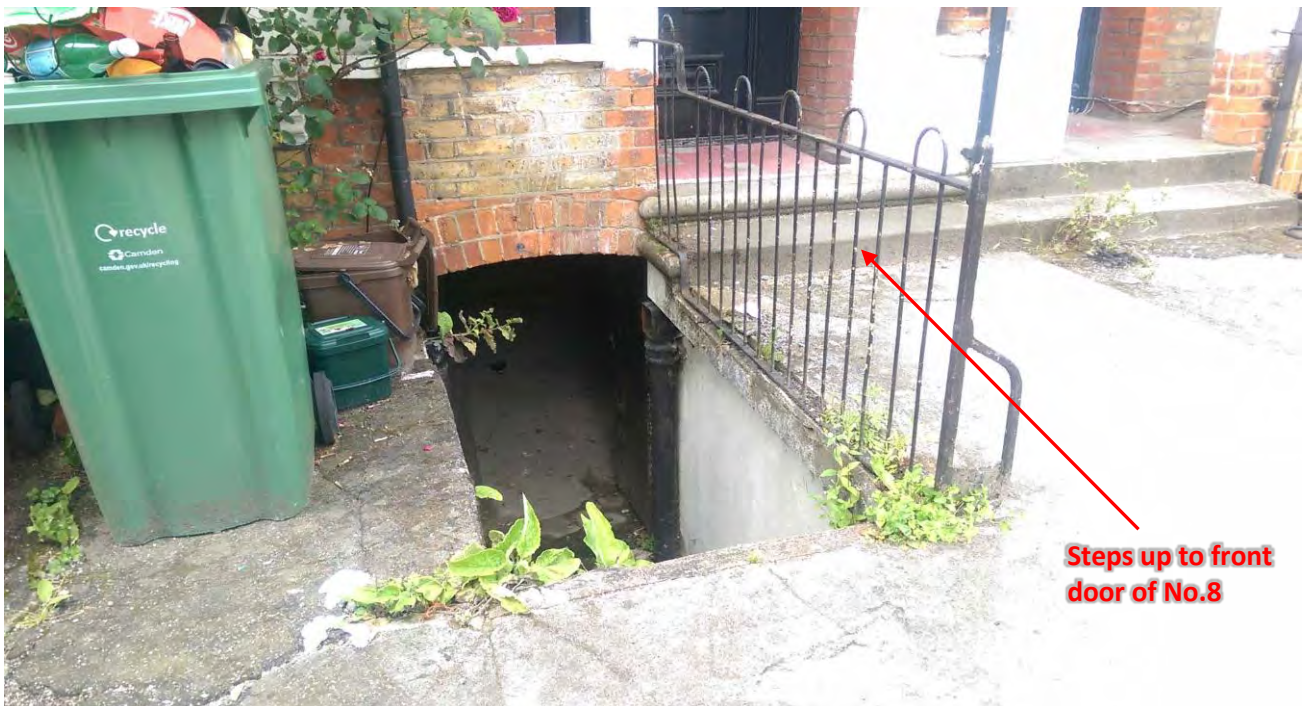
Photo 4: Access to the existing basement store is via external stairs only.
