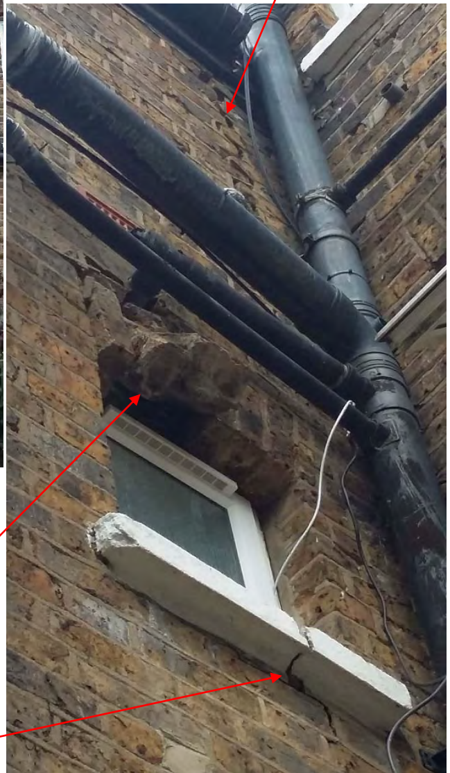
Severe instability of brickwork above first floor window
