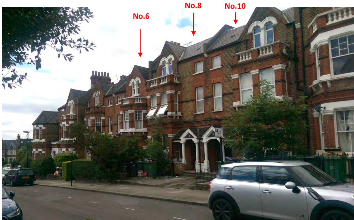
Photo 1: Front elevation, looking south. Note the consistent gentle southerly fall of the Agamemnon Road carriageway, and the change in level between No's 8 and No.6. Houses on Hillfield Road are visible at the extreme left of the photo.
