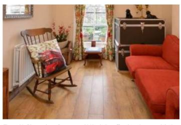
Figure 60: Photo taken of rear room 2013– timber effect boards over original floorboards. Skirting in this room appears to be later – it does not match that of the front room, which it would have done originally.
