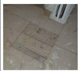
Figure 58: First floor hallway floorboards – appear to be original and have been retained.
