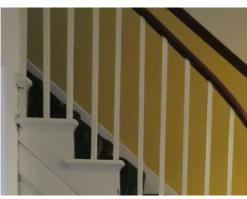
Figure 5: Simple timber balustrade on floor of lower hierarchy in a house of similar status and period.
