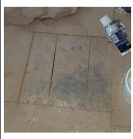
Figure 57: 1st floor – floorboards exposed – appear to be original and have been retained.
