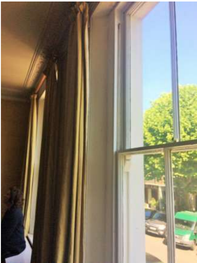
Figure 28: Detail of right hand window in Living Room. The lower sash is a later replacement.
