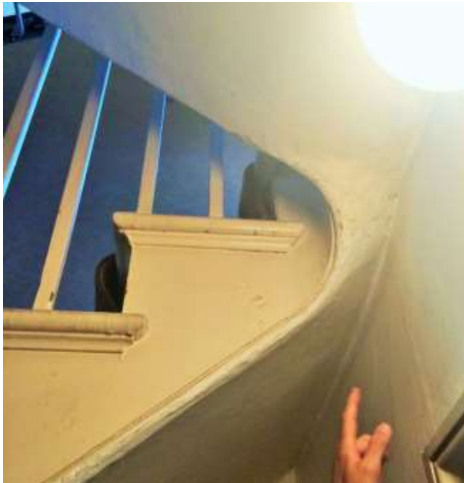
Figure 19: Wall between the back of the main house and closet wing abuts the curved underside of the staircase.
