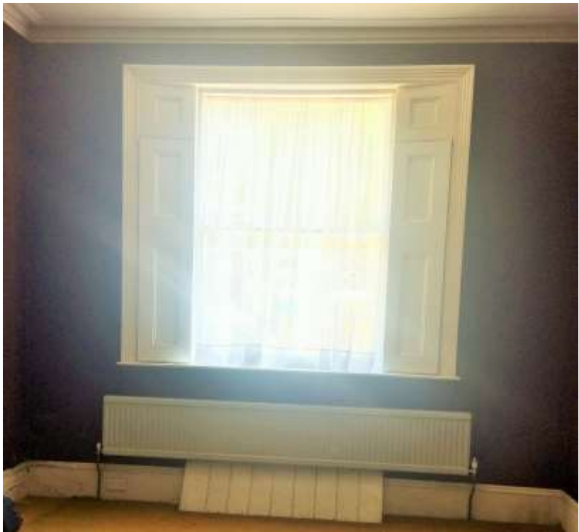
Figure 13: The window in Front Reception Room retain shutter boxes. The timber panelling under the radiator accommodates the tall window in Bedroom 1 of the Basement.
