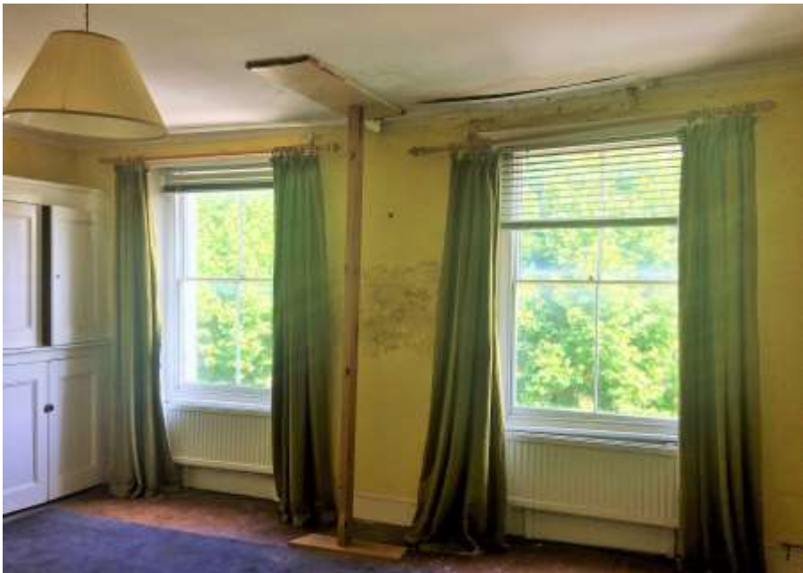
Figure 34: Front wall in Bedroom 3. The bottom sash of right hand window in Bedroom 3 has been replaced.
