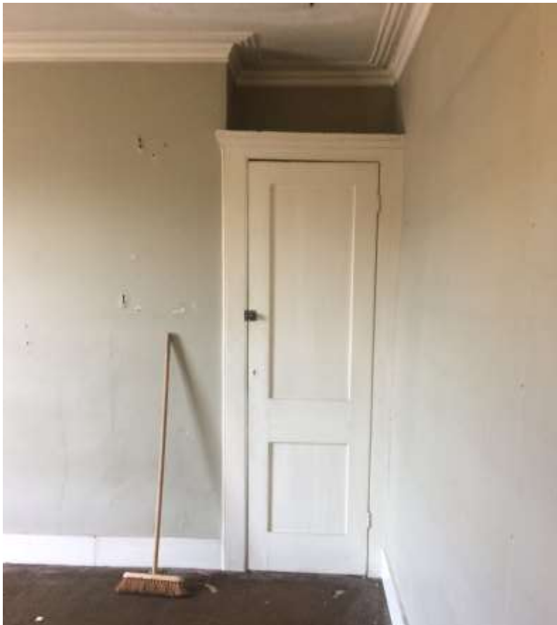
Figure 37: Chimney breast and built-in cupboard in side wall of Bedroom 4.
