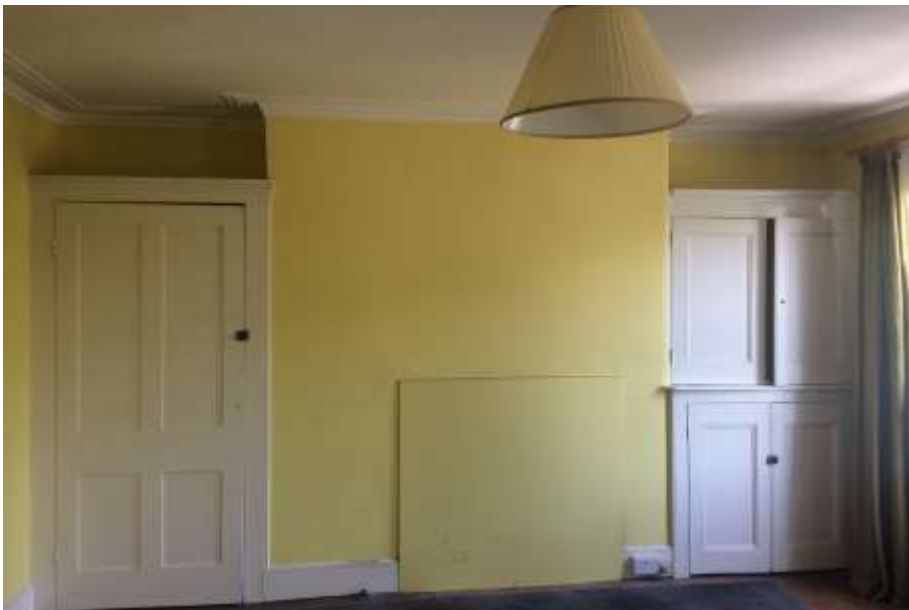
Figure 32: Side wall with chimney breast and two built-in cupboards in Bedroom 3.
