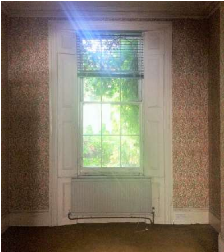
Figure 16: Original sash window and box shutters in the Rear Reception Room.
