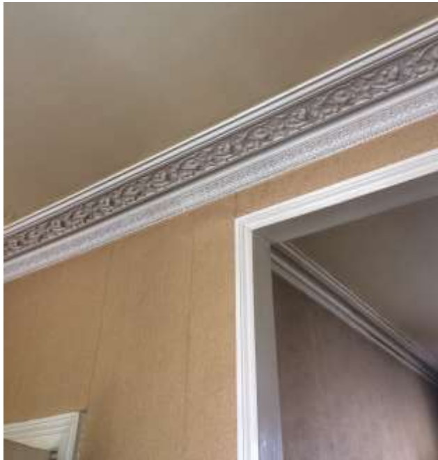
Figure 21: The cornice in the Living Room is more ornate than that in the Kitchen to the rear.
