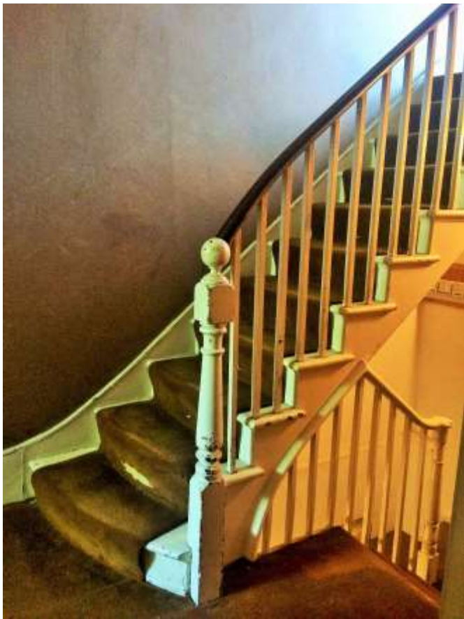
Figure 18: Staircase with probably original balusters.
