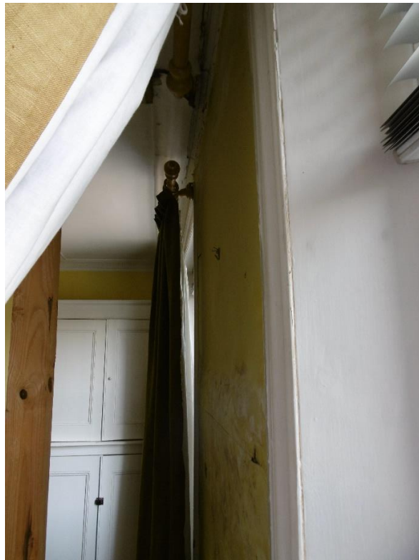
Photograph 6 - Bow to second floor front wall at roof level
