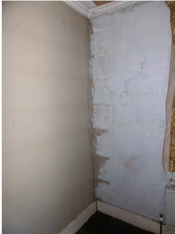
Photograph 7 - Cracking to cross wall with rear wall at second floor
