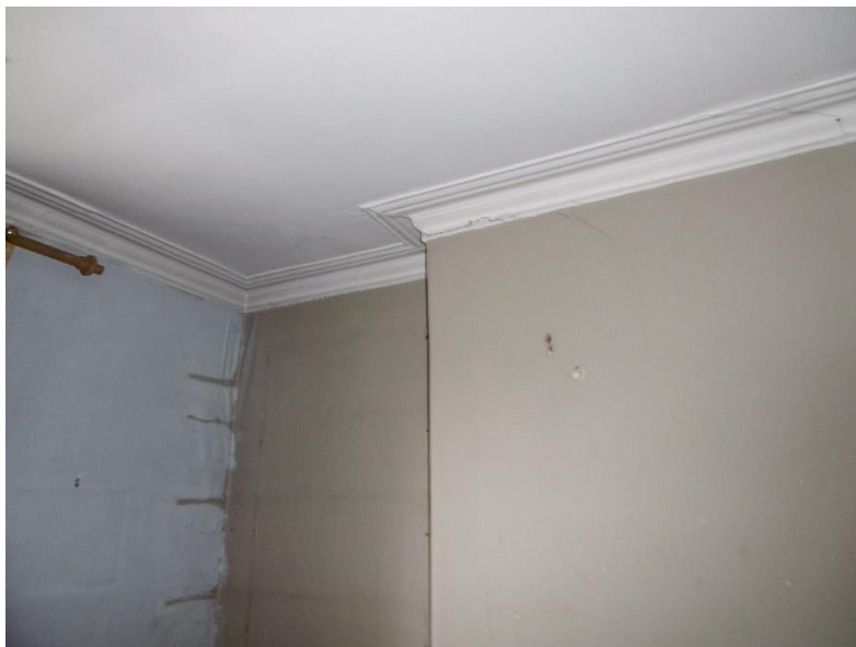
Photograph 8 - Cracking to ceiling and party wall at rear wall
