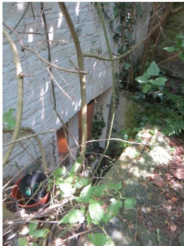
Photograph 12 - Bow to rear extension basement wall and cracking at render
