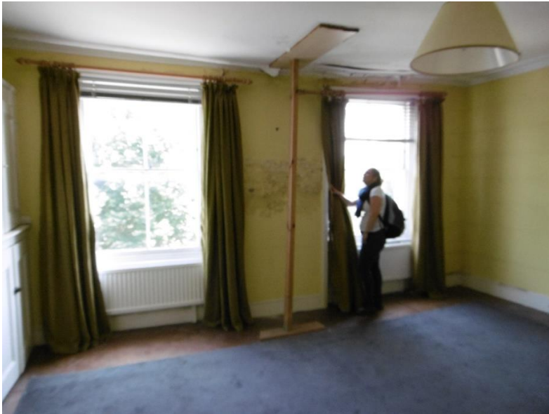
Photograph 5 - Second floor front bedroom ceiling propping
