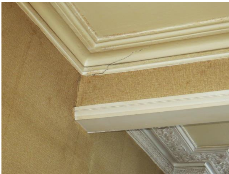
Photograph 10 - Cracking to first floor opening around lintel bearing
