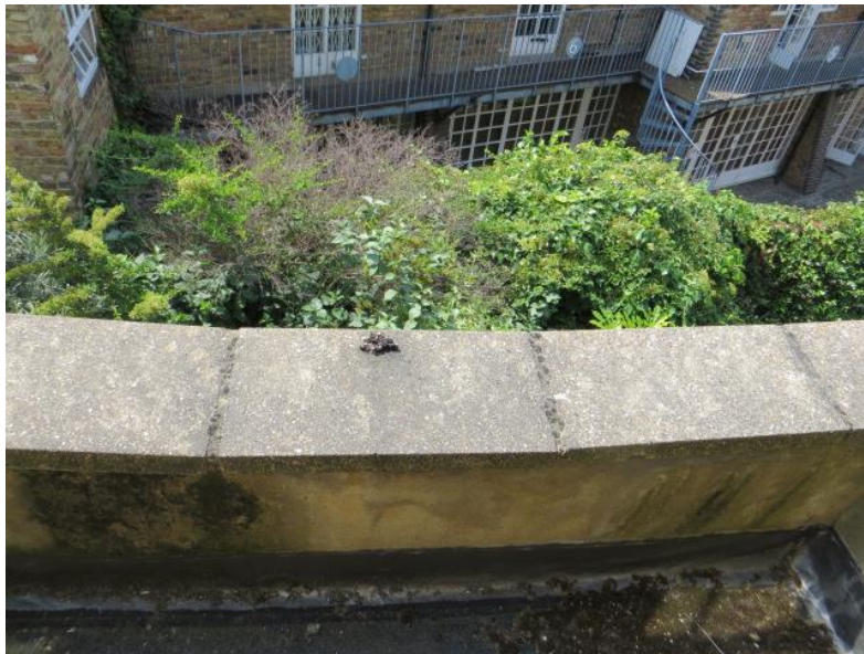
Photograph 11 - Bow to parapet showing no sign of cracking
