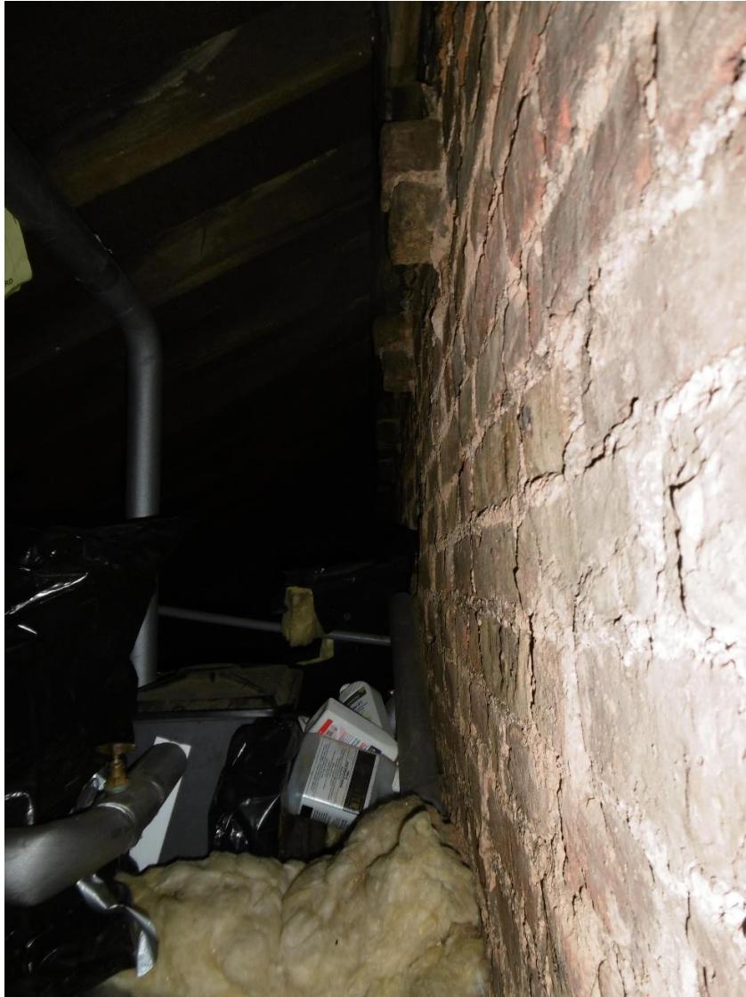
Photograph 13 - Rafters to butterfly roof supported on corbels on party wall
