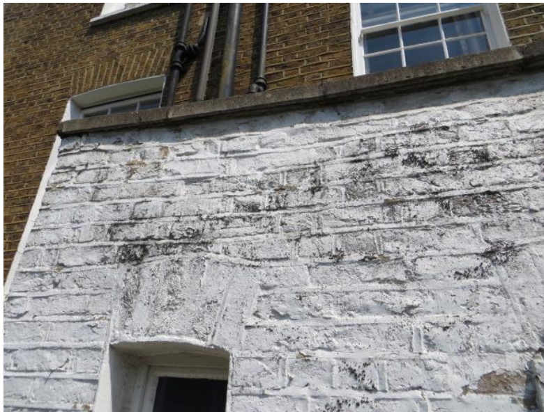
Photograph 3 - White latex paint to rear extension causing damage to brick faces
