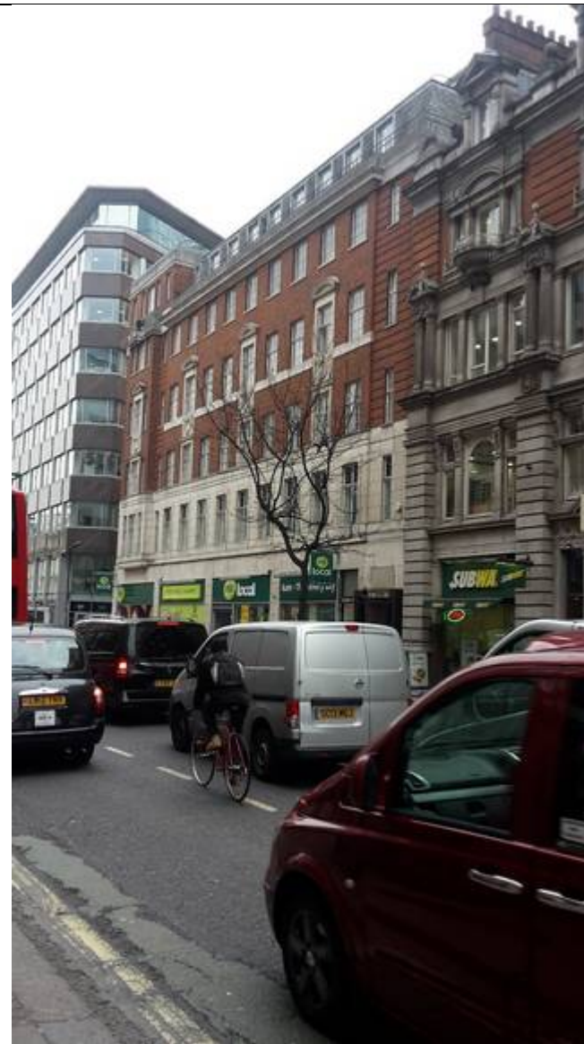
Plate 4: Medius House frontage from New Oxford St.
