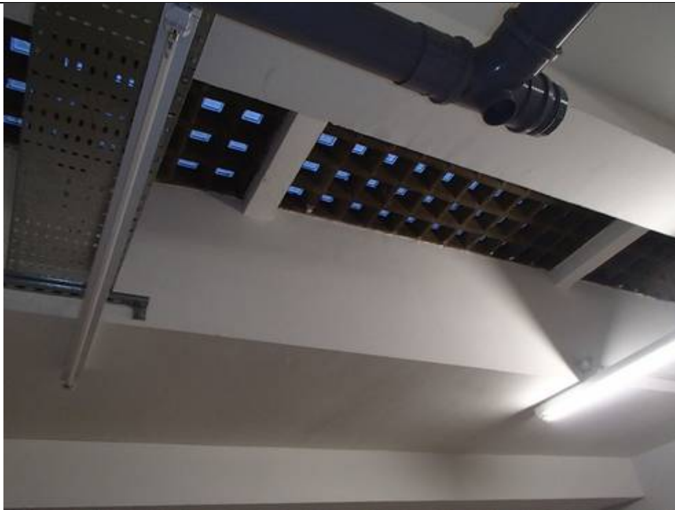
Plate 5: Basement lightwell, Medius House.
