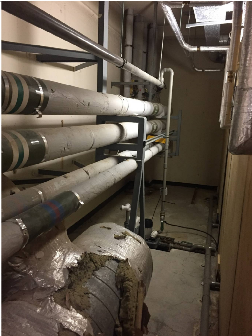
Plate 7: Internal service corridor, Castlewood House.
