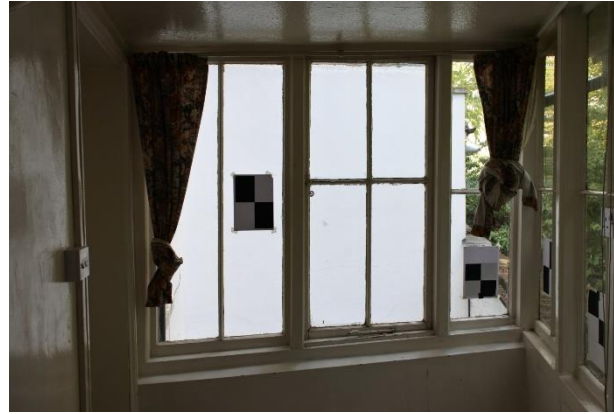
Ground Floor Kitchen in rear extension
