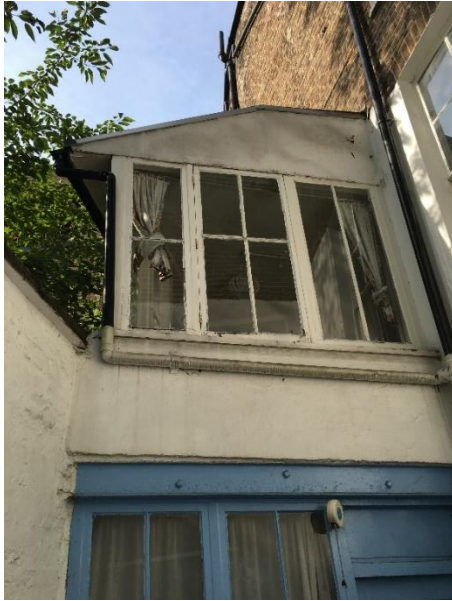
Ground Floor rear extension to be demolished
