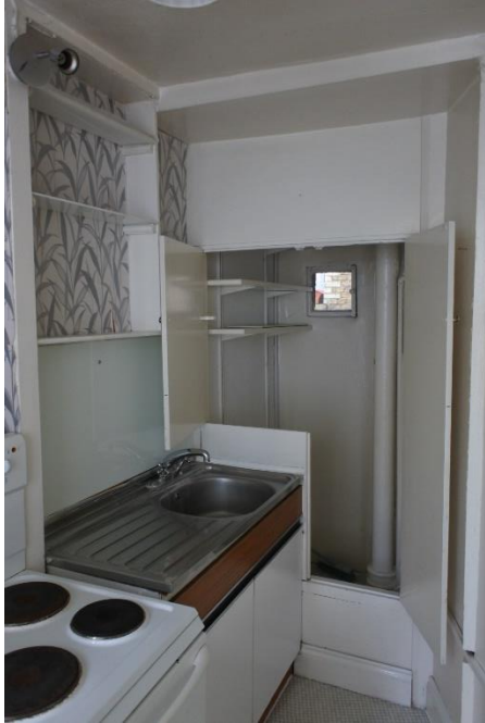
Ground Floor Kitchen in rear extension
