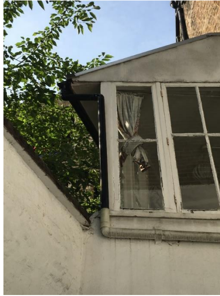
Ground Floor rear extension to be demolished
