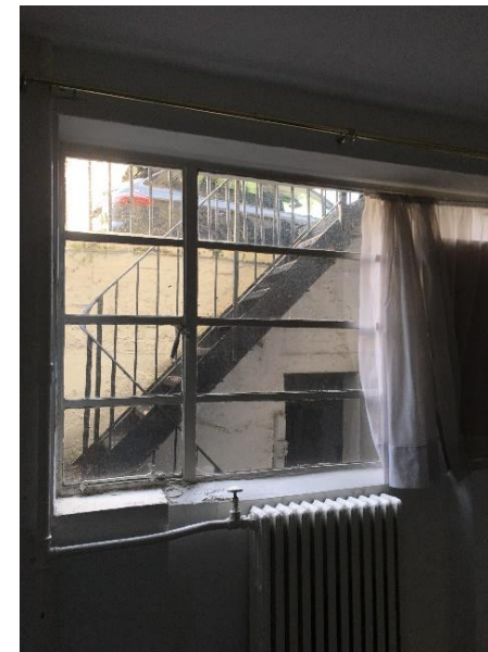
Front bedroom window showing metal stairs and vault beyond
