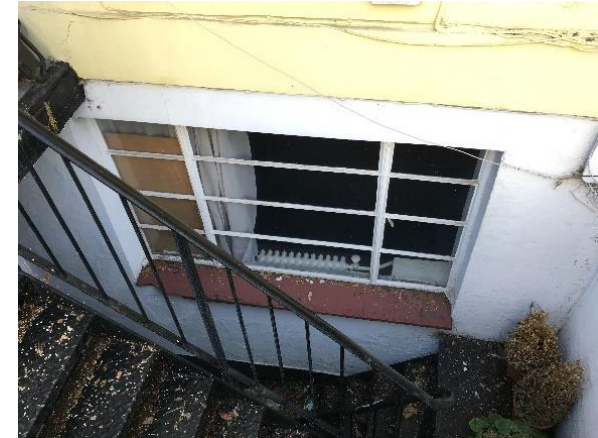
Front bedroom window and metal stair
