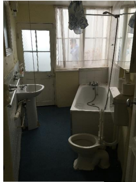
Bathroom showing external door
