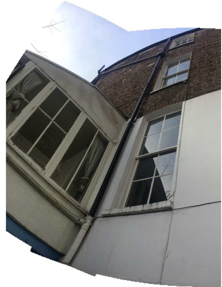
View up from lower basement terrace
