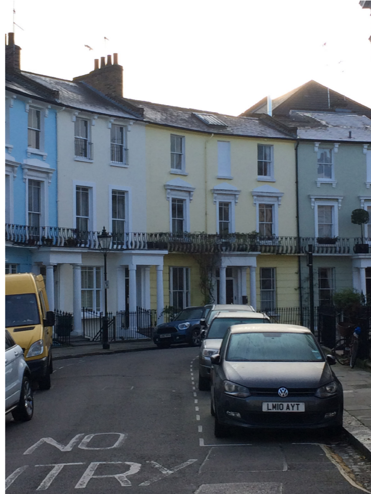
View east along Chalcot crescent, no 26 painted yellow
