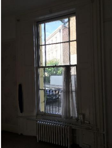
Ground Floor bedroom front window
