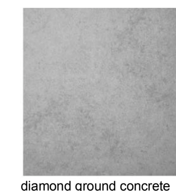
diamond ground concrete
