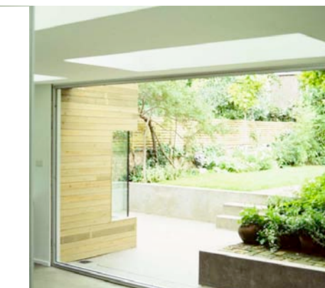
sliding doors to kitchen and dining area NB: slim profile black steel frames
