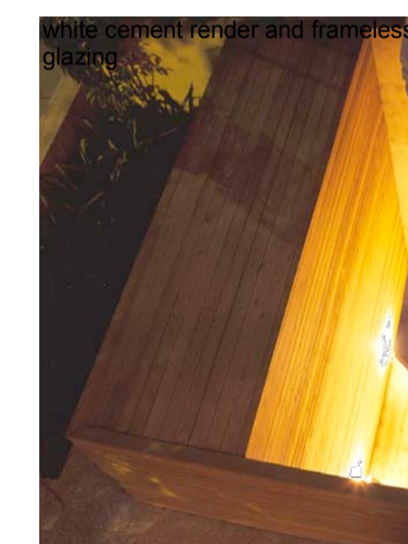
lightwell with timber cladding
