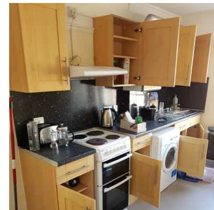
16 - Existing low quality kitchen units
