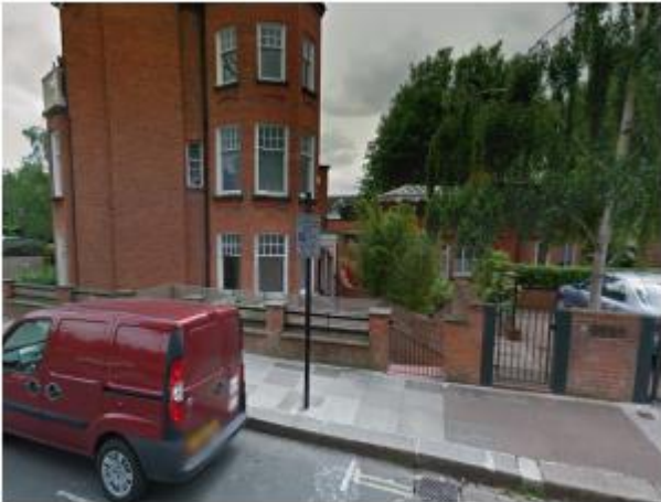
LOCATION B WITHOUT POLE
