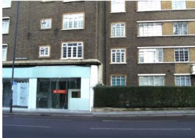
LOCATION B WITHOUT POLE
