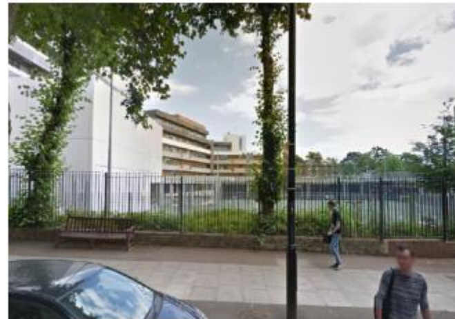
LOCATION B WITHOUT POLE
