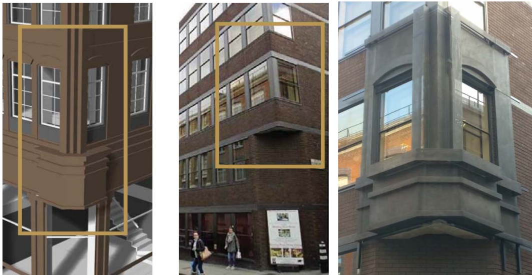
Figure 5: Sample panel location on computer model and existing building, and sample panel in position.
