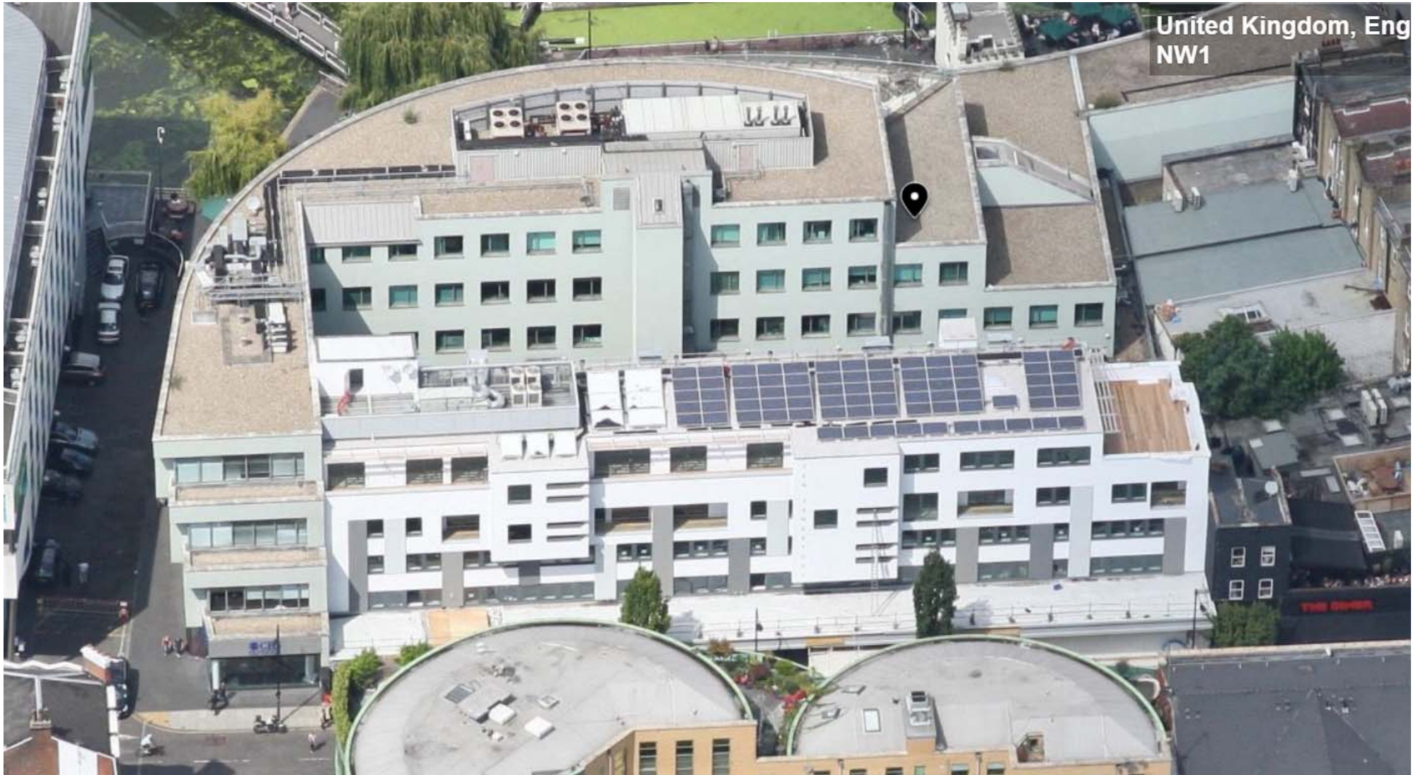
Aerial view of south elevation
