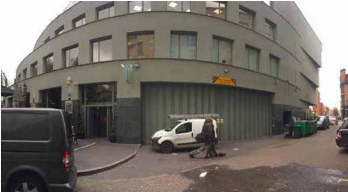
View of existing service yard entrance
