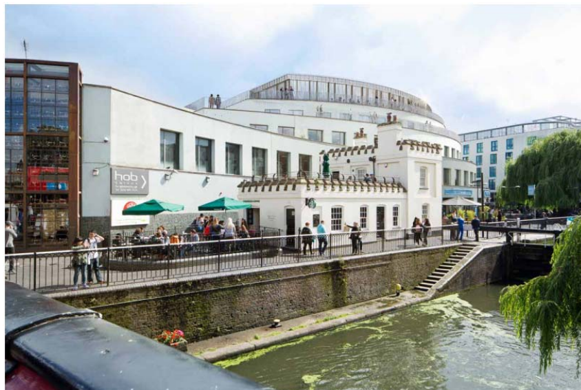
Figure 4 – The proposed site viewed from Camden High Street
