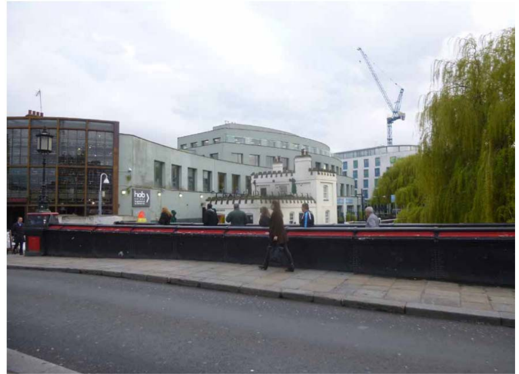
View of the existing building from Chalk Farm Road
