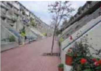
The strong architectural character means that it appears the least changed. The 'red brick' paving and waterproofing have been completely re-laid with about 60% new paviors, because of the breakdown of the waterproofing layer and problems with cast-in conduits and expansion joints, the brick paving and water proofing.<sup>66</sup>
