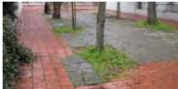
Mix of concrete paving and red pavers in very poor condition lifted around trees (this area was used as a contractor's compound during recent building works). *Robinias* in mixed ages/sizes and condition. Planters with ivy growing up flank walls.
