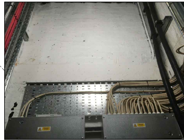
Riser to be above existing distribution board
