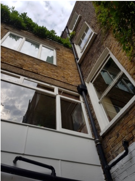
View of existing rear wing from light well
