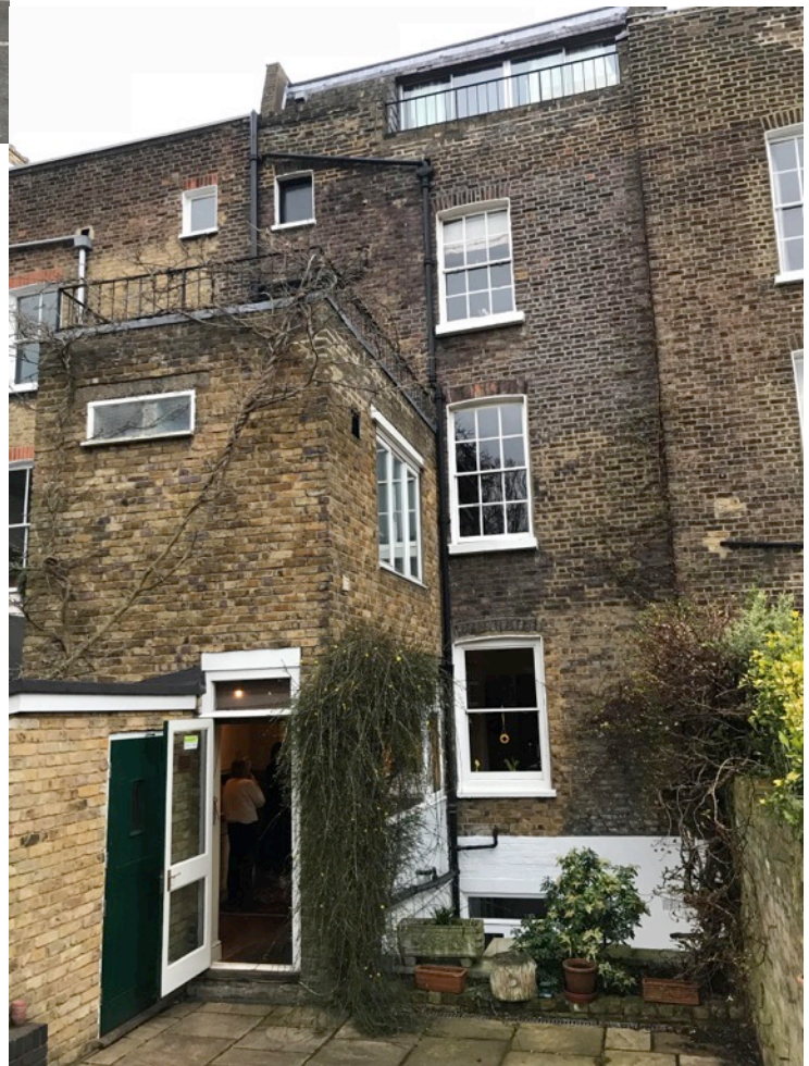
View of existing rear facade from garden
