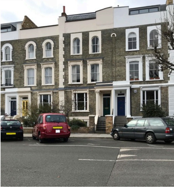
View of existing front façade from roadside
