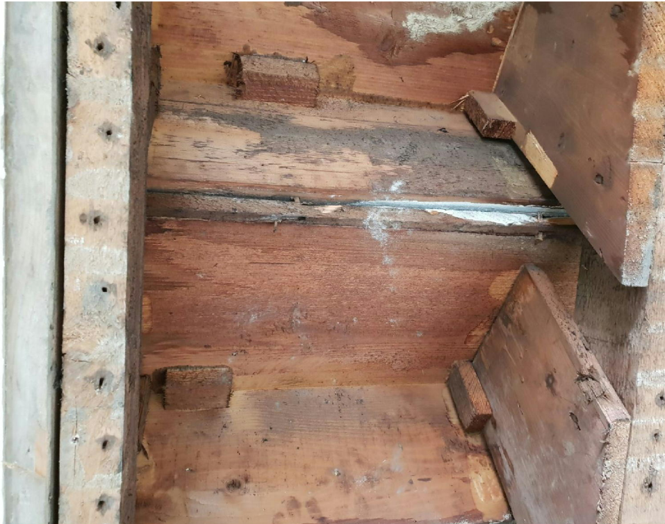
PHOTOGRAPH 3: first to second floor flight
