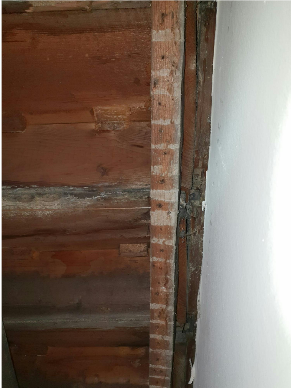
PHOTOGRAPH 4: first to second floor flight
