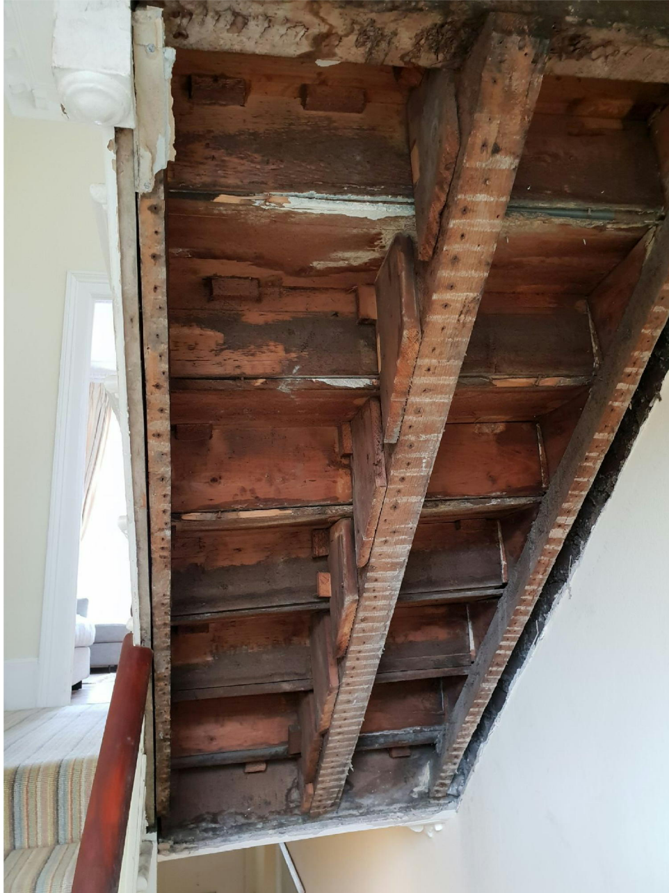
PHOTOGRAPH 2: underside of flight, lathe & plaster removed
