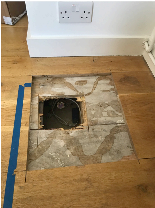
Third Floor- Existing Floor Materials- 18mm non-original floorboards / 18mm plywood
