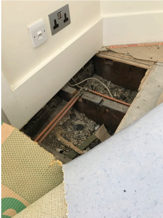
Second Floor- Existing Floor Materials- carpet / 18mm chipboard
