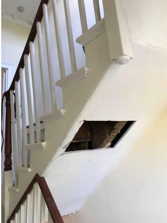
Stairs First floor to Second floor
