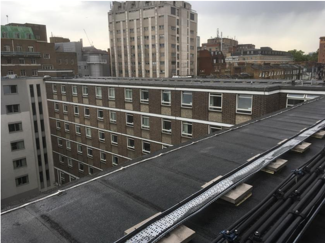
Photo of existing roof
