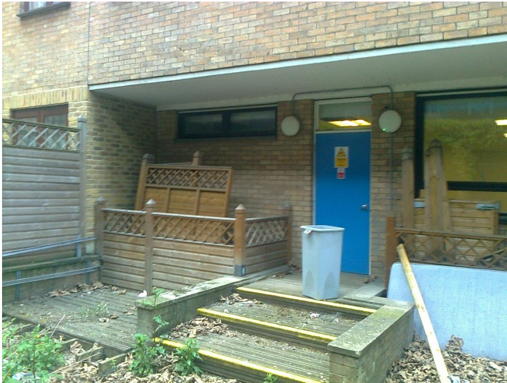
7. Existing rear ground floor elevation of 4 Tavistock Place
