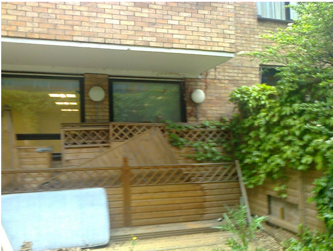
8. Existing rear ground floor elevation of 4 Tavistock Place
