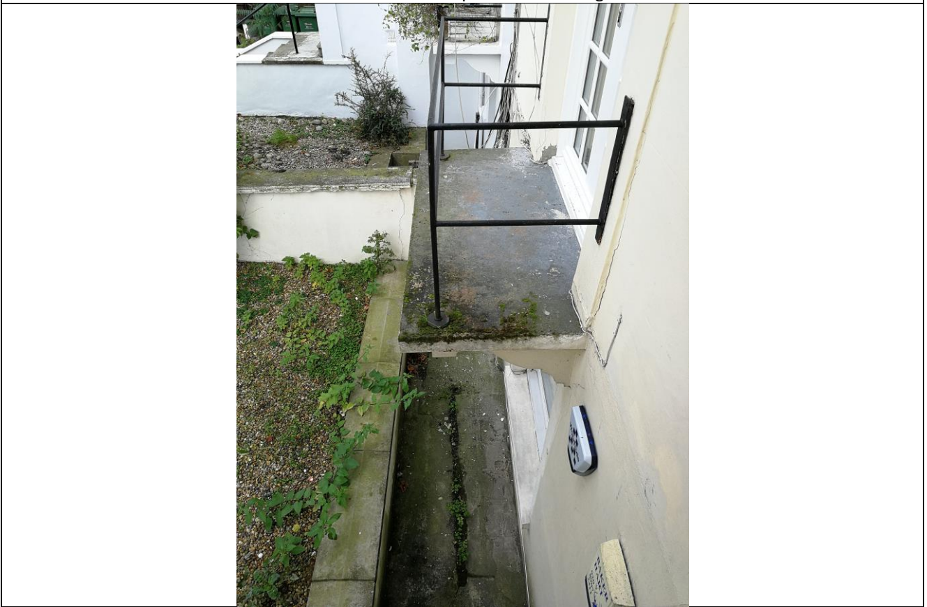
Photo 5 – First Floor projecting balcony railings
