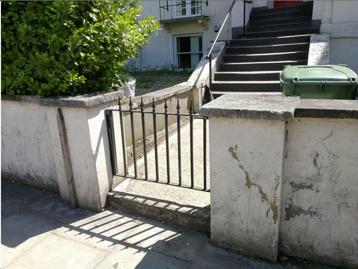
Photo 2 – Entrance gate and front boundary wall
