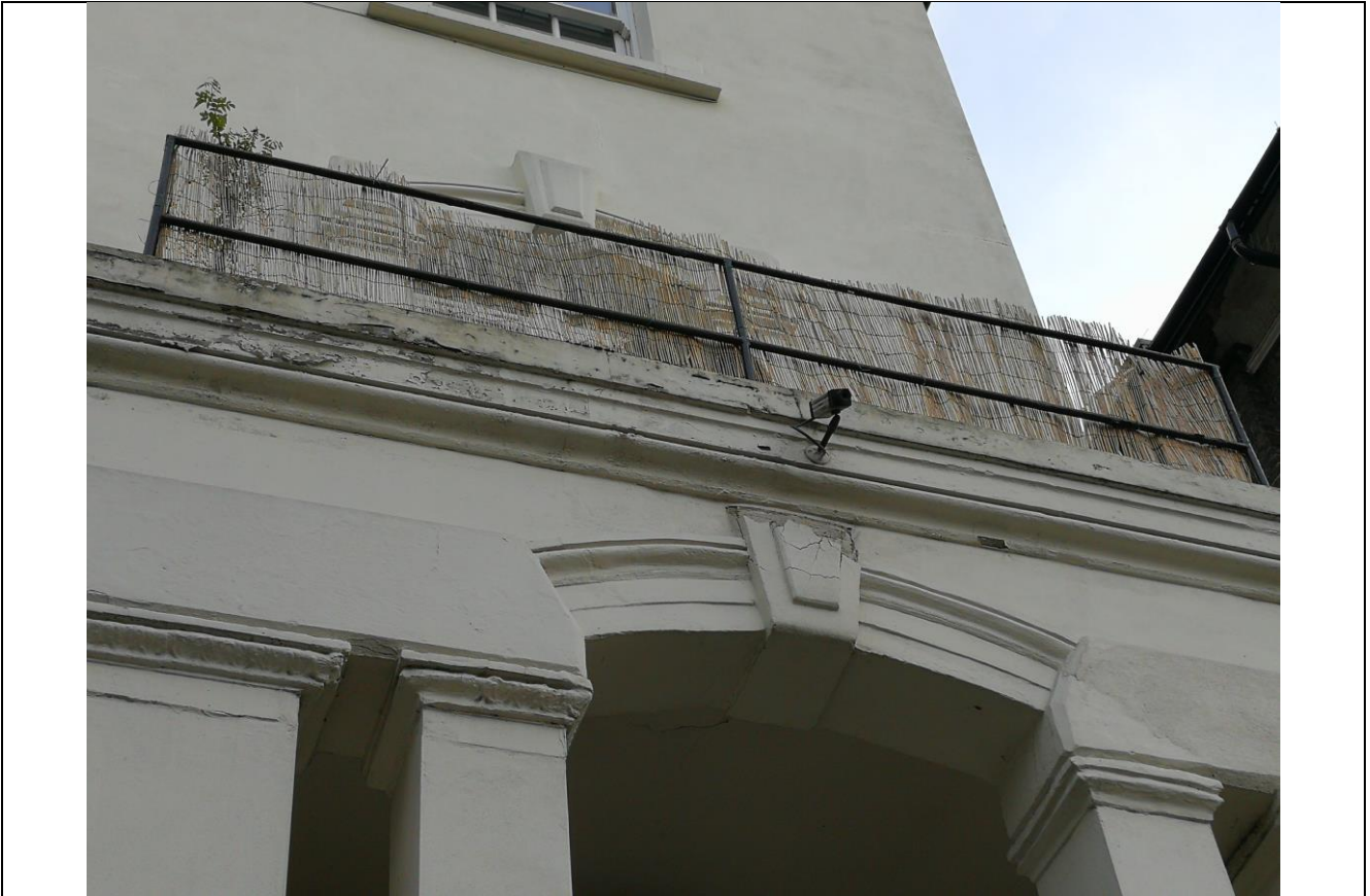
Photo 4 – Entrance porch metal railings
