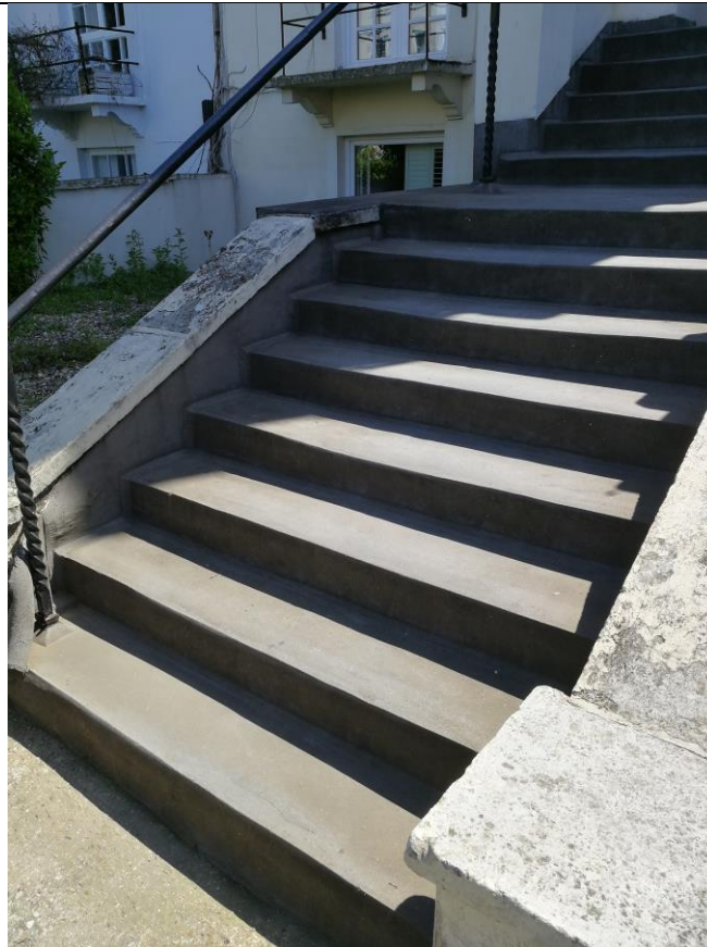
Photo 3 – Existing asphalt covering to steps and metal handrail
