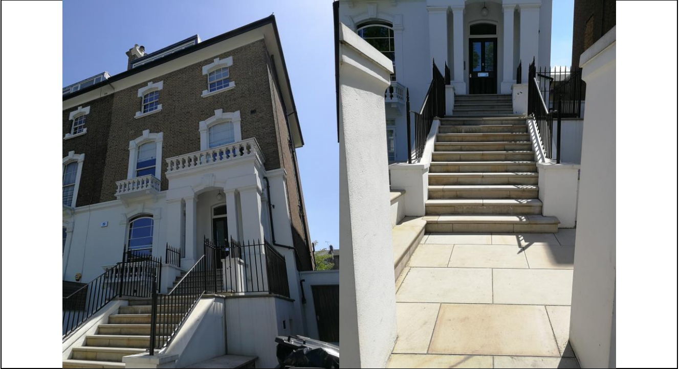
Photo 10 – Adjacent property entrance steps and railings, to be replicated. No.236 Camden Road.
