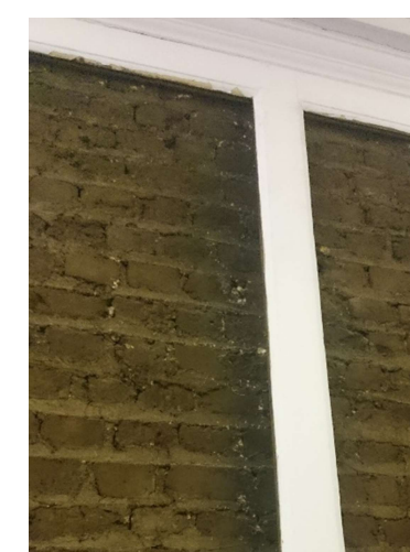
Figure 11. Typical solid brick wall at basement
