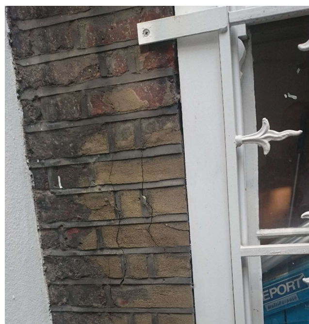
Figure 15. Hair line cracking to front elevation
