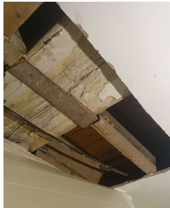
Figure 6. Typical timber joists and transfer beam
