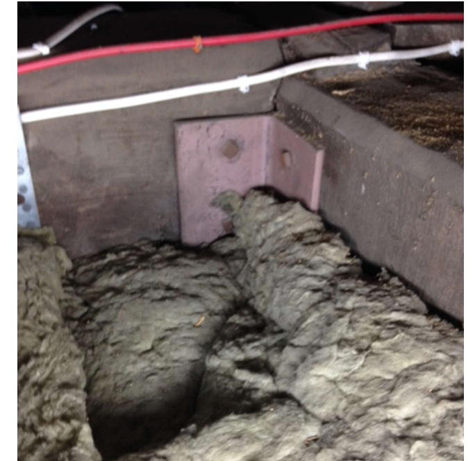
Figure 9. Typical timber loft transfer beams
