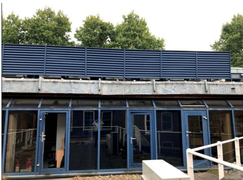
Figure 20 Plant screen above Jockeys' Field with existing condensers
