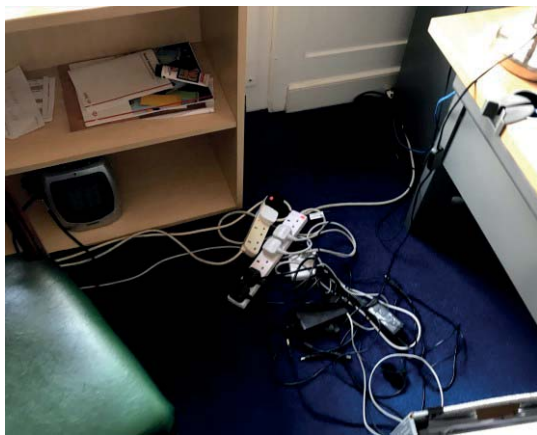
Figure 10 Typical cables tangle due to existing floor boxes being in wrong location
