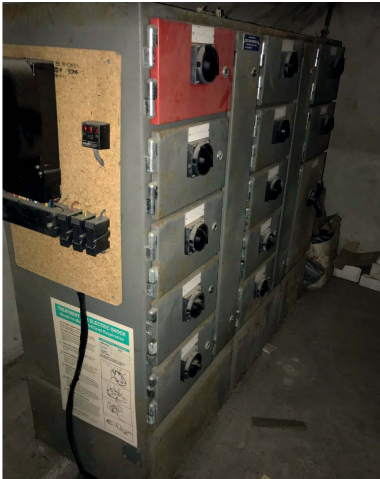
Figure 2 Electrical meter and LV panel at Bedford Row to be re-used
