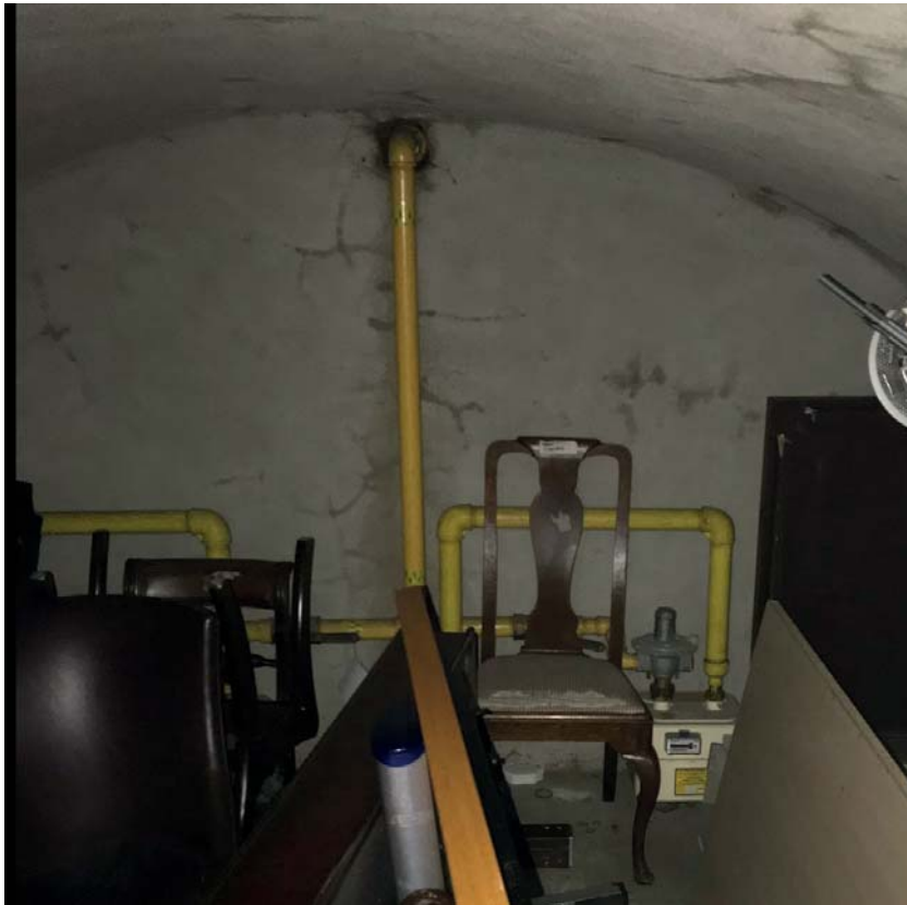
Figure 3 Gas meters at Bedford Row to be stripped
