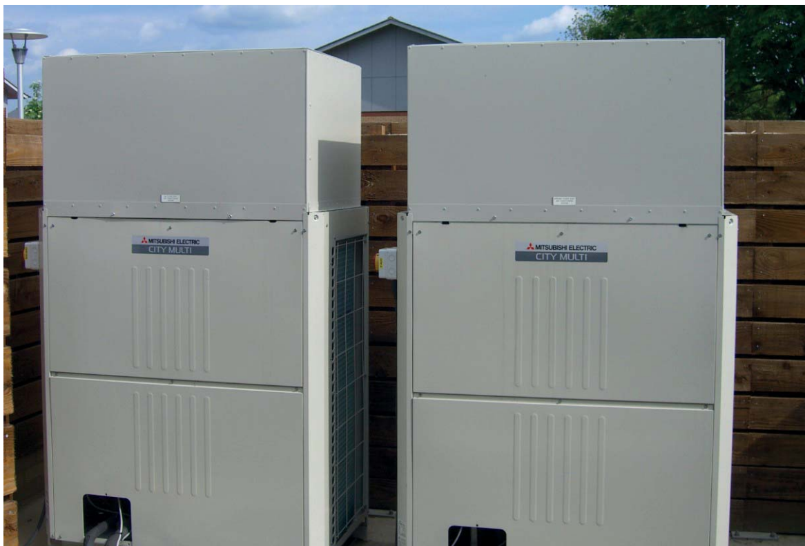
Figure 23 Typical discharge attenuators
