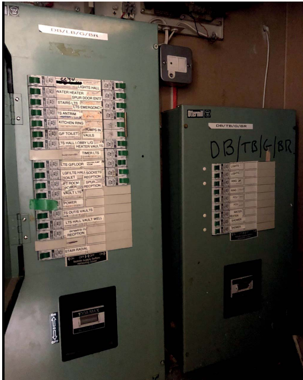
Figure 6 Existing distribution board at LG Bedford Row
