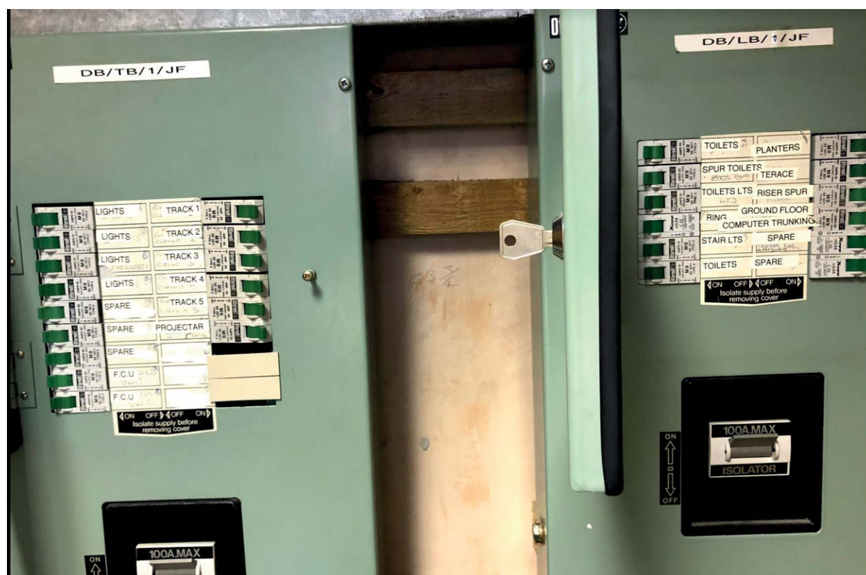
Figure 5 Existing Jockeys' Field boards 10 Way capacity
