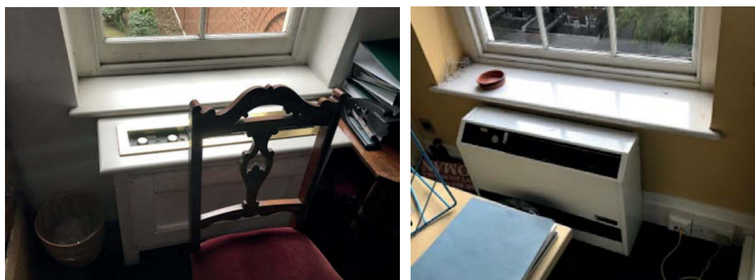
Figure 26 Existing fan coils intrude into the space.
