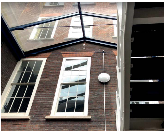
Figure 13 The existing Atrium Beam detection will be re-used
