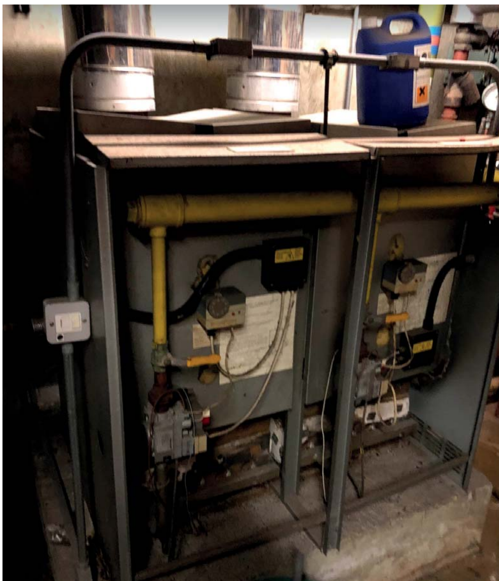
Figure 4 Existing Gas supply to boilers in Jockeys' Fields enters from west of plant area.
