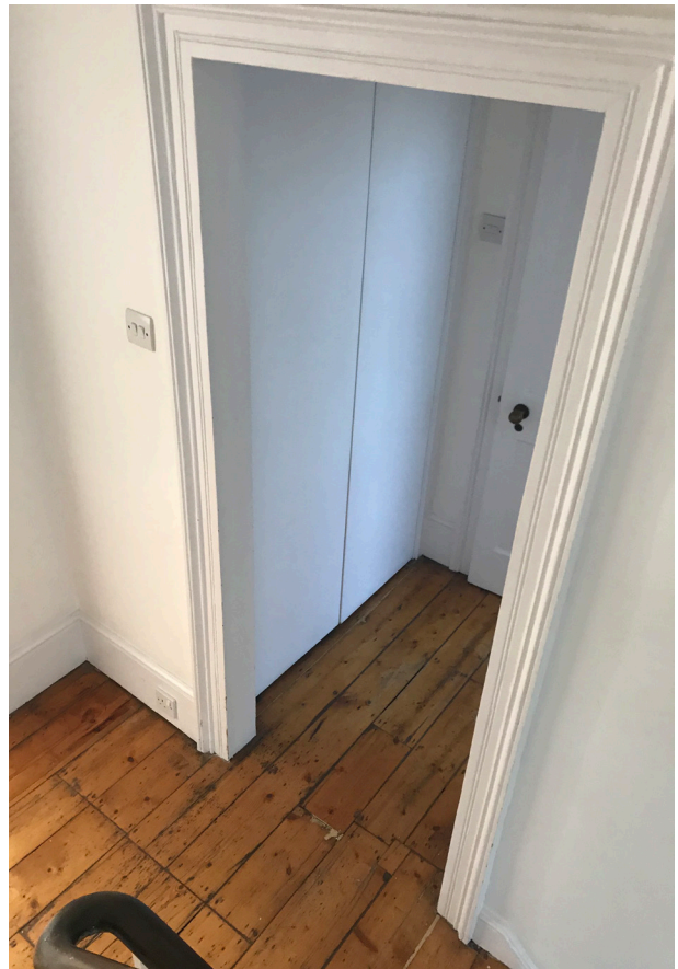
Original covings, skirtings and architraves to be retained or replicated throughout Original timber floor boards to be retained and reused as necessary to work with new layouts
