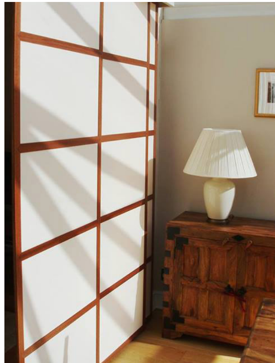
Example of type of lightweight partition proposed for third storey bedroom
