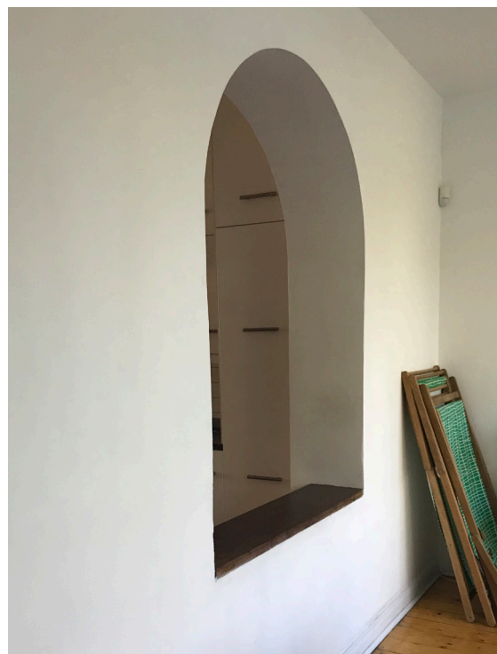
Non-original arched opening between kitchen and sun room which difficulties movement through the ground floor
