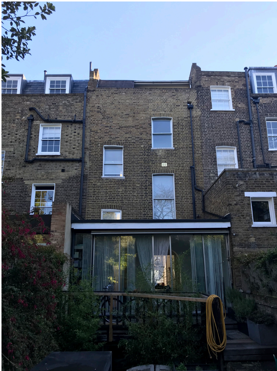
View of rear elevation showing low quality single storey ground floor extension, and non-traditional sash windows to upper floor
