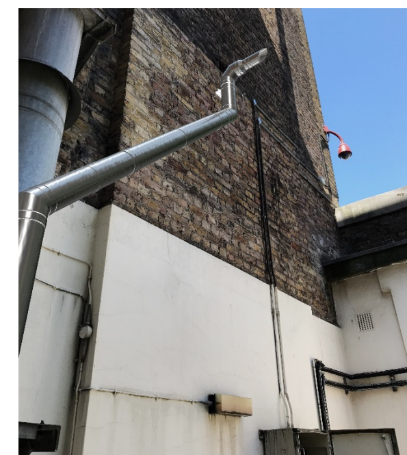
Fig 2: 1a Montague Street Proposed Flue Installation
